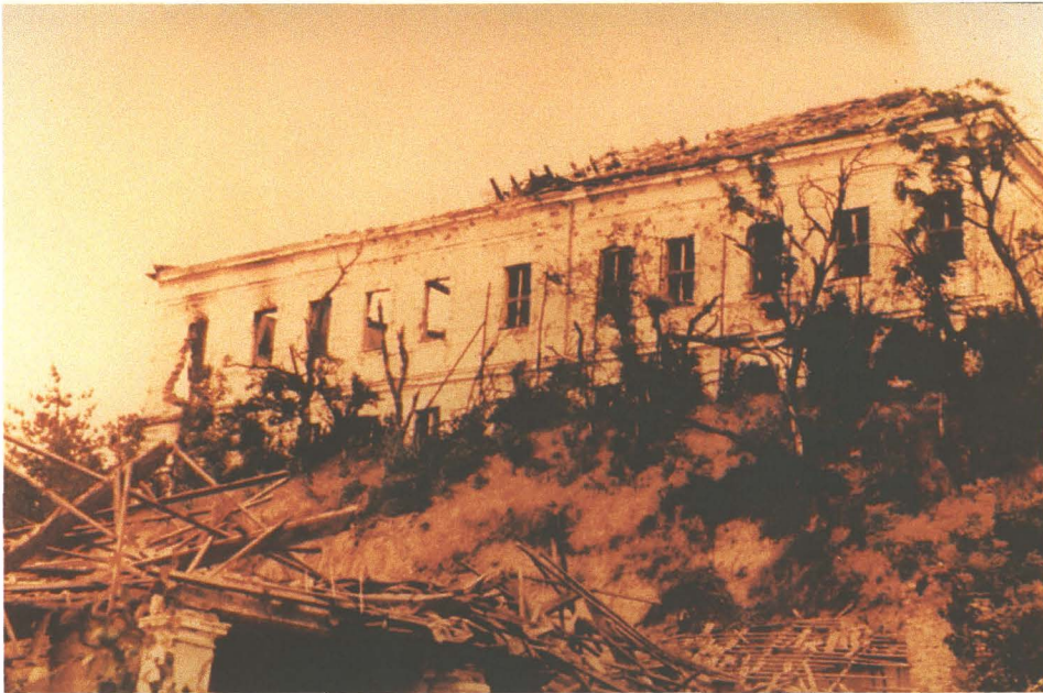
12.1 REMNANTS OF VUKOVAR GRAMMAR SCHOOL BUILDING AFTER SEVERAL MONTHS OF SHELLING
