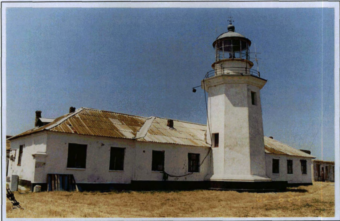
Photo D: The Lighthouse Complex in 2002 before Reconstruction
