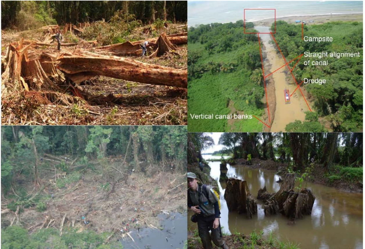
Figure 3.4: Image comprising several photos included in the records which evidence the damages caused by the clearing of trees and vegetation and dredging of C2010 and CE2013. Source: Figure 11 to Neotrópica Report, Annex 1
