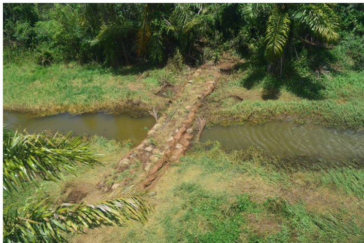
Photo 13. Final condition of the area where the dyke was built. Photo by Miguel Araya, 6 April 2015.
