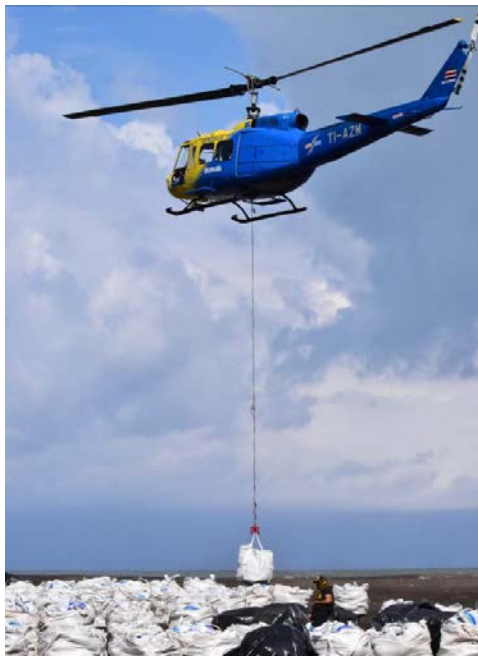
Figure 3.6: Photographs of The civilian helicopter being used to transport sacks of sand and deposit them in the 2013 eastern caño , 3 and 4 April 2015.
