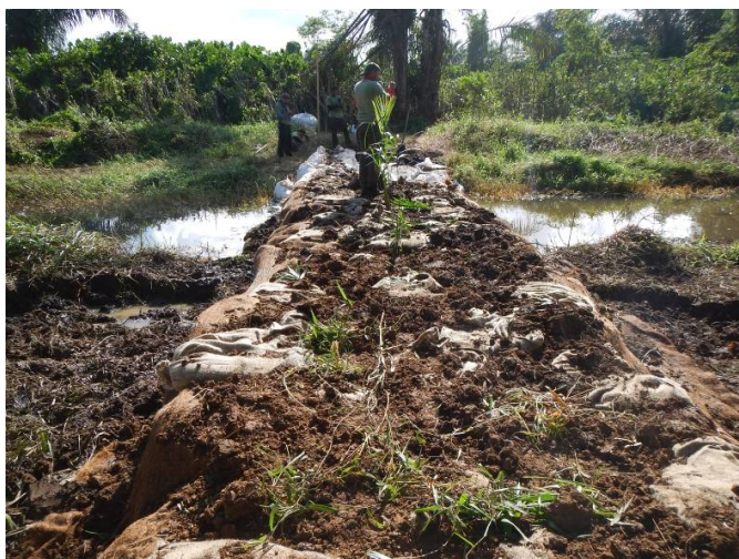
Photo 11. Covering of the dyke with material present at the site, result of the dredging. Planting over the dyke. Photo by Miguel Araya, 6 April 2015.
