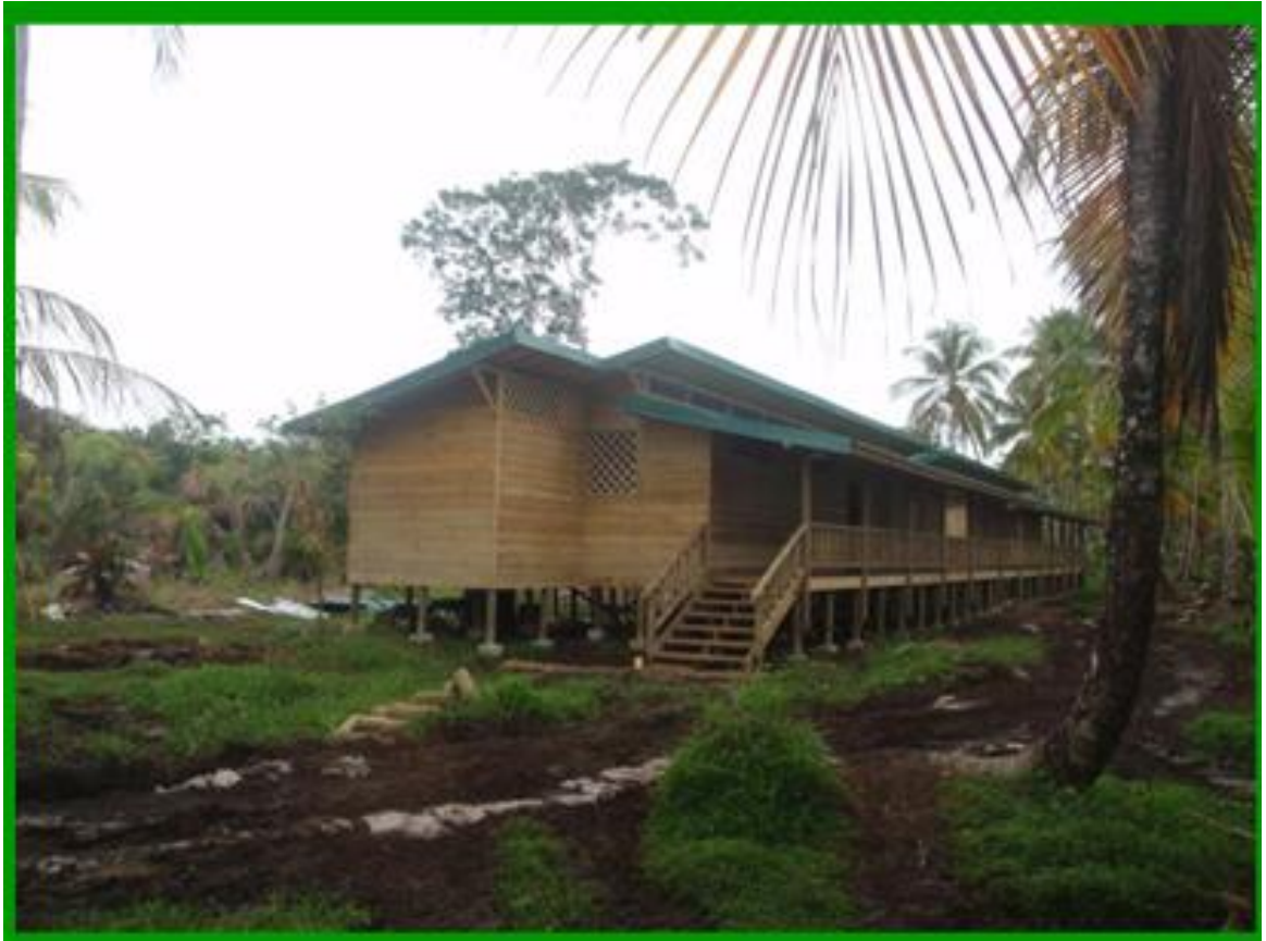
Figure 11: Photograph of the side of the MINAET biological station
