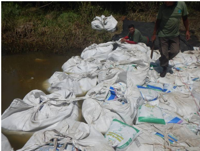
Photo 8. Arrangement and tying of sacks. Photo by Olman Mena, 2 April 2015.
