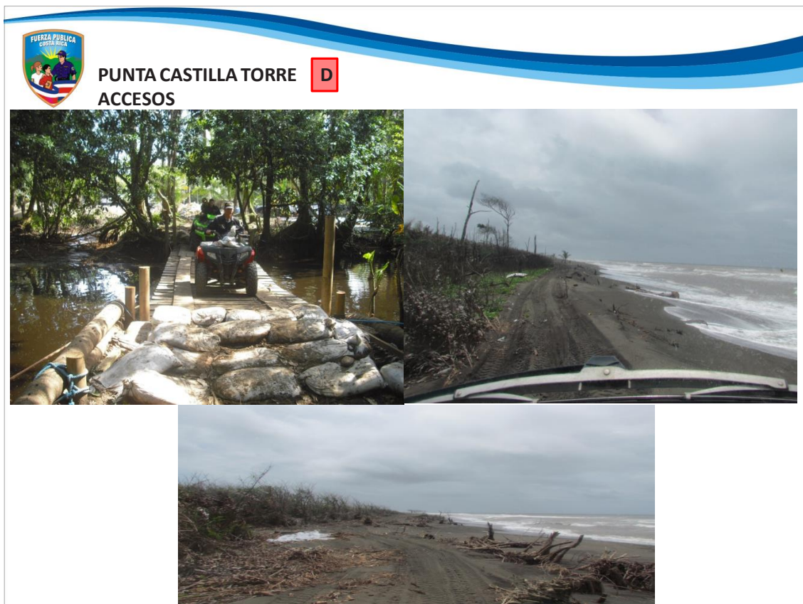
Figure 8: Access to police post and Tower D at Punta Castilla
