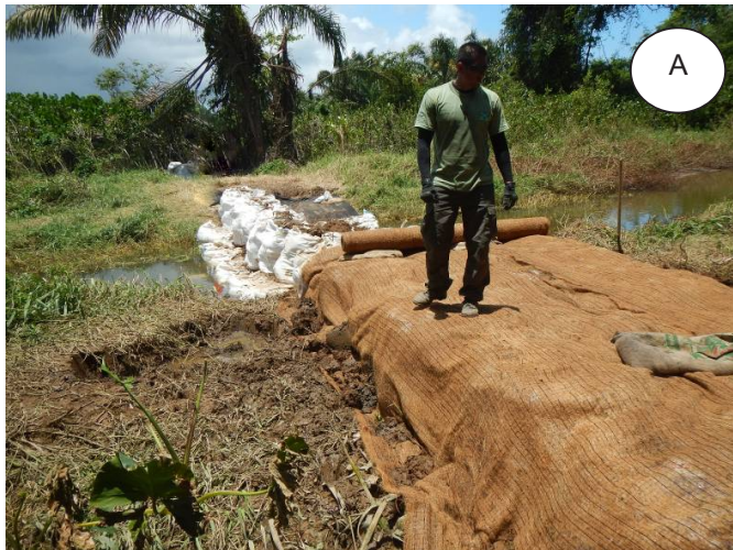
Photo 9. Coconut fibre laid out over the sacks (A) and burlap sacks placed to set the coconut weaved textile. Photo by Miguel Araya, 6 April 2015.
