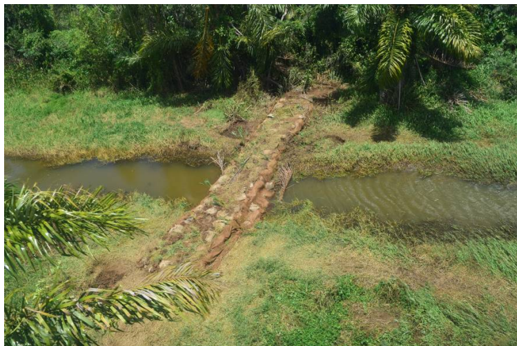
Photo 13. Final condition of the area where the dyke was built. Photo by Miguel Araya, 6 April 2015.
