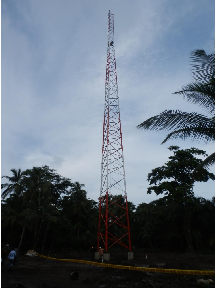
Figure 10: Tower D at Punta Castilla
