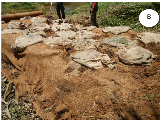
Photo 10. Partial view of the coconut fibre setting process using natural fibre sacks, and placement of soil in surrounding areas. Photo by Miguel Araya, 6 April 2015.
