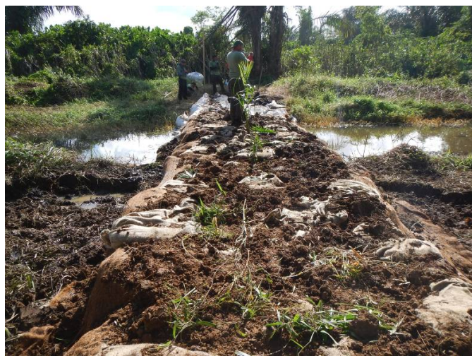
Photo 11. Covering of the dyke with material present at the site, result of the dredging. Planting over the dyke. Photo by Miguel Araya, 6 April 2015.
