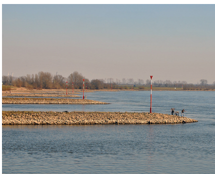
Figure 3: Typical lowland river (Waal) with groynes.
