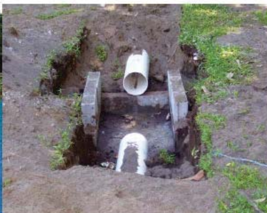
Photo No. 6. Drainage Pipe.
