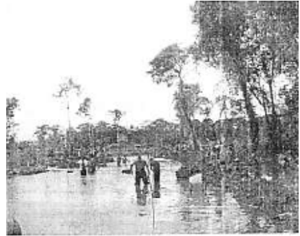
Beginning of the manual clearing
