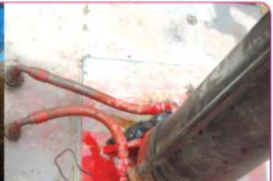
"SOBERANÍA I" hydraulic cylinder oil leak
