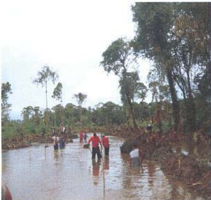
Manual cleaning work
