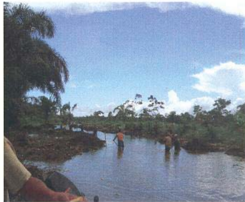
Manual cleaning work
