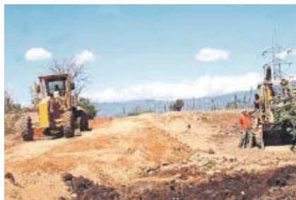
route 1856, Juan Mora Porras, under construction.
