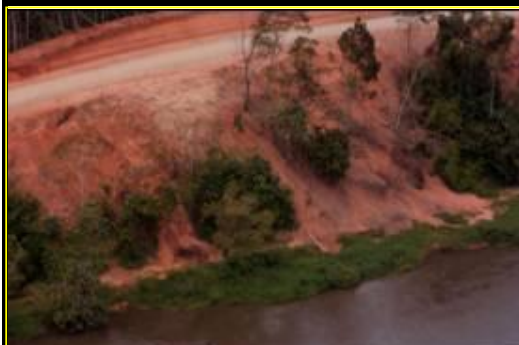
Figure 37: Critical point due to slope instability and ongoing erosion process
