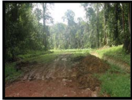
F12. Dirt roads where water has accumulated making transit impossible. Impact on the forest can be observed.
