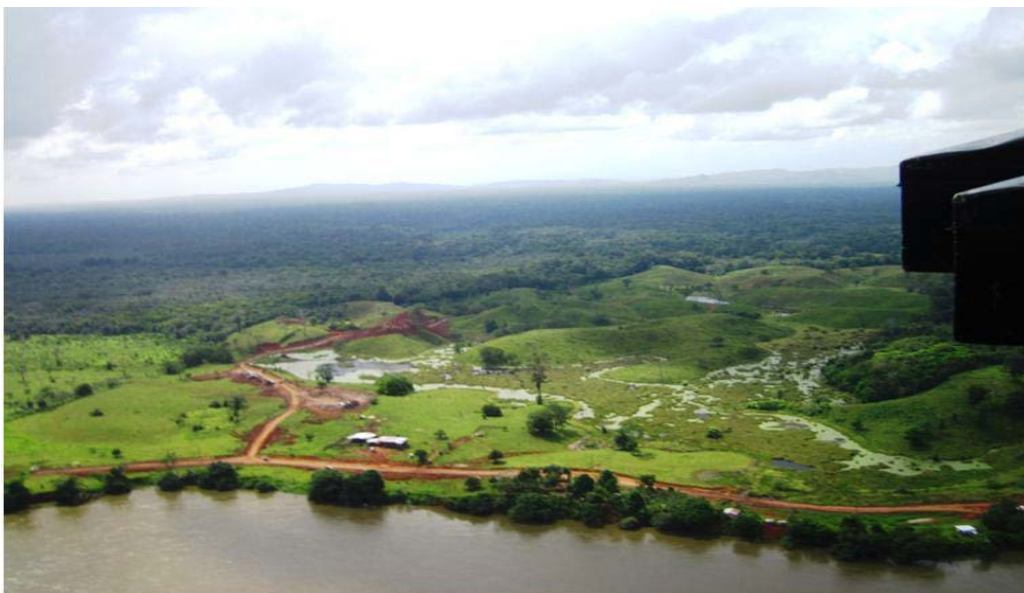
Figure 53: Plant and wildlife destruction caused by road construction
