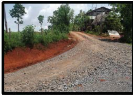
F38. Dirt road from Route 760 El Parque.
