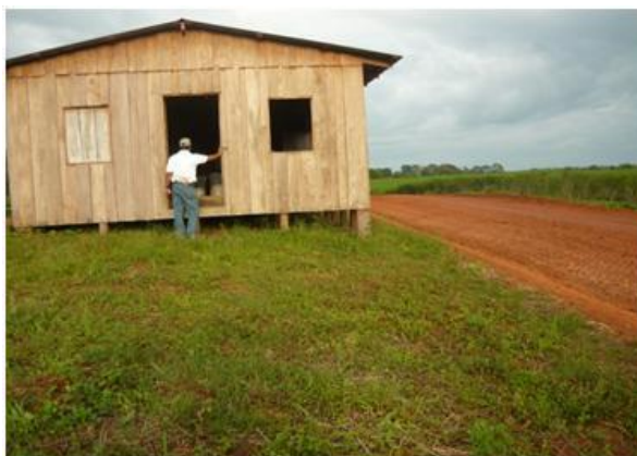
Figure 12: Dwelling at edge of road slope
