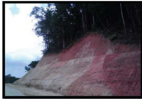
F.28. There are huge slopes with high peaks in this area and no protection whatsoever.
