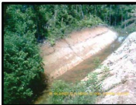
F52. Dirt drainage ditch serving as water outlet.
