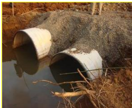
Figure 10: Culverts located on Nicaraguan territory
