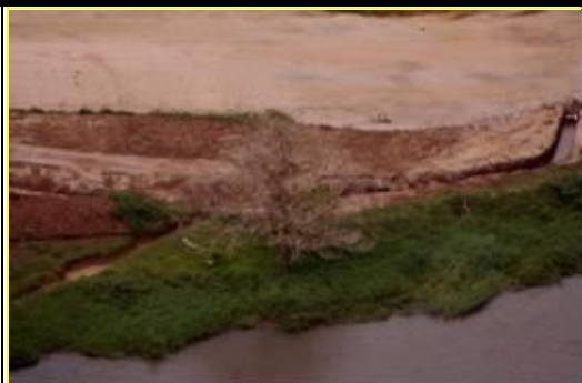
Figure 38: Critical point due to silting in the river channel
