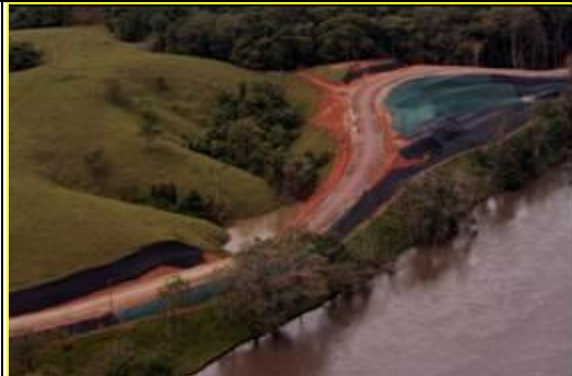
Figure 40: Critical point due to slope instability
