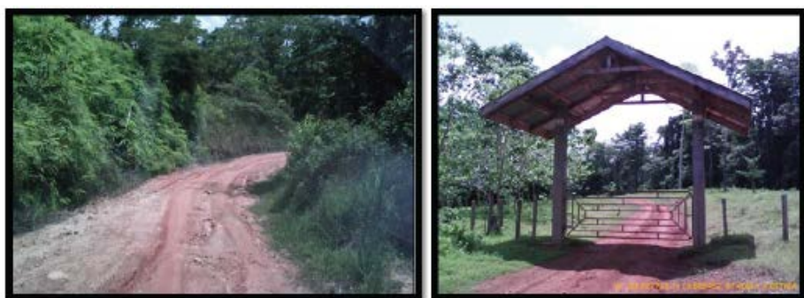
F24. Areas with cracks and holes and no drainage.
