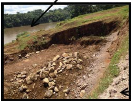
F19. Materials used are only meters away from the Río San Juan; very big boulders can be observed as well as piles of broken boulders. Here, what is apparently a trench is located between the Río San Juan and the road, several meters from the river. These situations should be evaluated.
