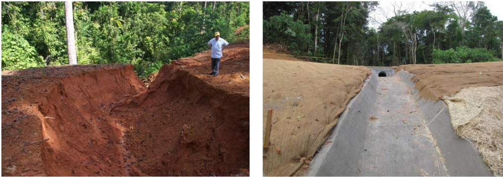
Figure 40. View down a large gully in a fill prism created by concentrated runoff from the Road draining to Costa Rican territory to the west of Marker II (a) in February when it was actively eroding and (b) in May when the gully had been back-filled and stabilized using a culverted cross-drain and concrete drainage channel, with coconut matting used to protect the surrounding fill slope from sheet and rill erosion. Photographs by the author.
