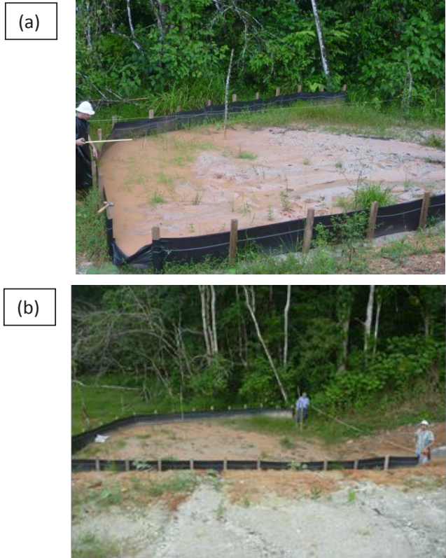
Figure 29. Sediment trap #2 on (a) 8 June and (b) 22 July 2013 (from the UCR Report).
