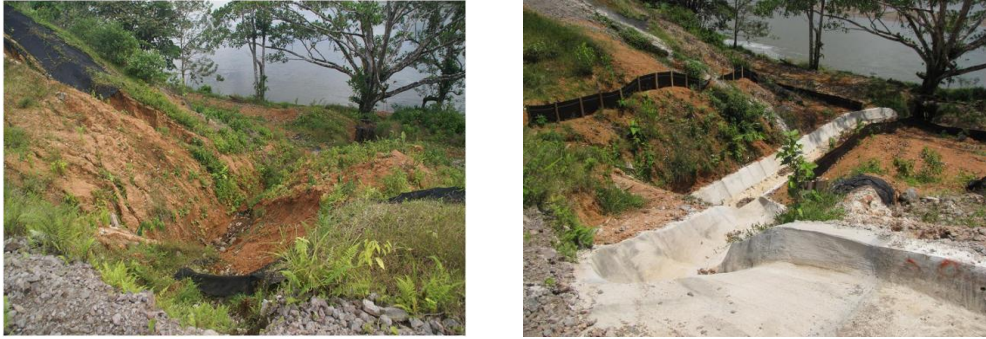
Figure 42. Road at East 498072, North 325345, about 6.6 km east of Marker II (a) on 15 February 2013 showing a network of gullies on an outboard slope and sediment accumulated as a run-out deposit on the flat terrace surface separating the foot of the slope from the bank of the Río San Juan (b) on 7 May 2013 showing mitigation works in the form of concrete channels and drop structures to convey runoff from the road bed, and silt fences to protect the slope from sheet and rill erosion, lined out-board and prevent road-derived sediment reaching the terrace. A sediment trap had also been constructed at the downstream termination of the gully system to prevent sediment reaching the River, though this cannot be easily identified in the photograph. Photographs by author.
