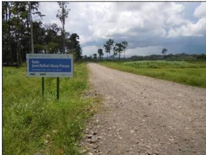
Figure 2. Condition of platform in road section 1.
