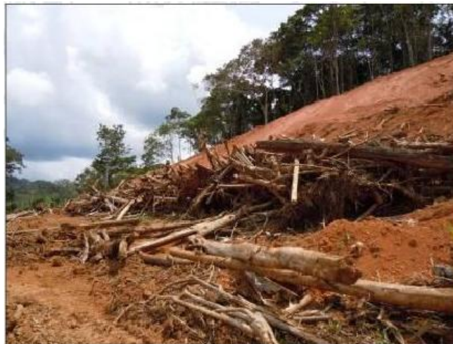
Figure 29. Brush and tree trunks laid at embankment foot, road section 6. Source: LannameUCR, May 2012
