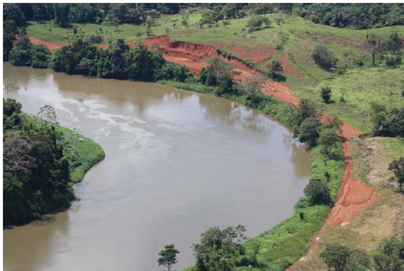
Figure 9. Photo #121b at km 39.0 from upstream end of Route 1856 along border. Route 1856 has been constructed well within 50 m of the Río San Juan. Note the extensive surface erosion along the road, as well as large cutbank landslides, the poorly constructed stream crossing in the middle right, and the lack of any erosion control or wet-season stabilization efforts.
