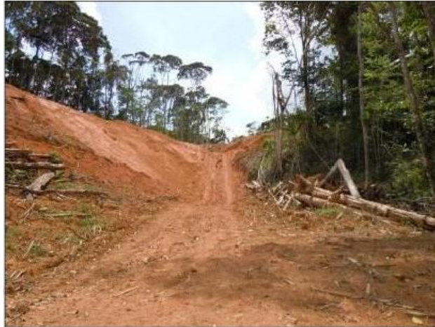
Figure 28. Fill area, road section 6. Source: LannameUCR, May 2012
