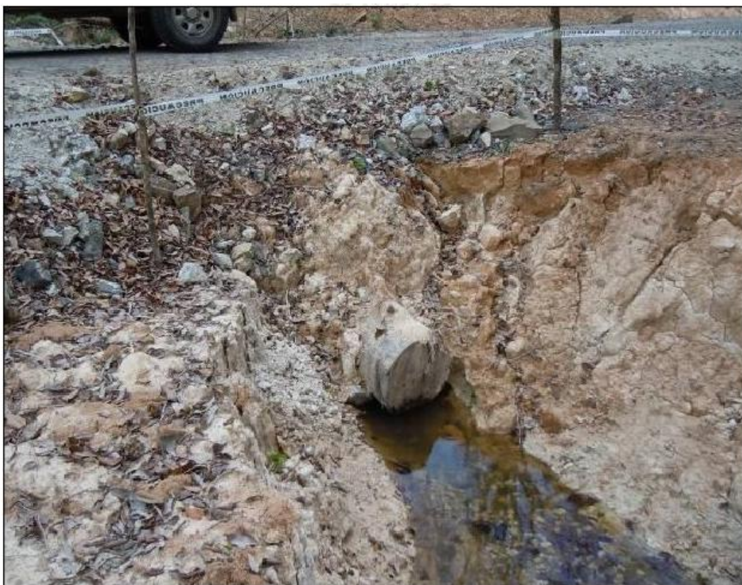
Figure 34. Logs used for stream crossing in road section 7.
