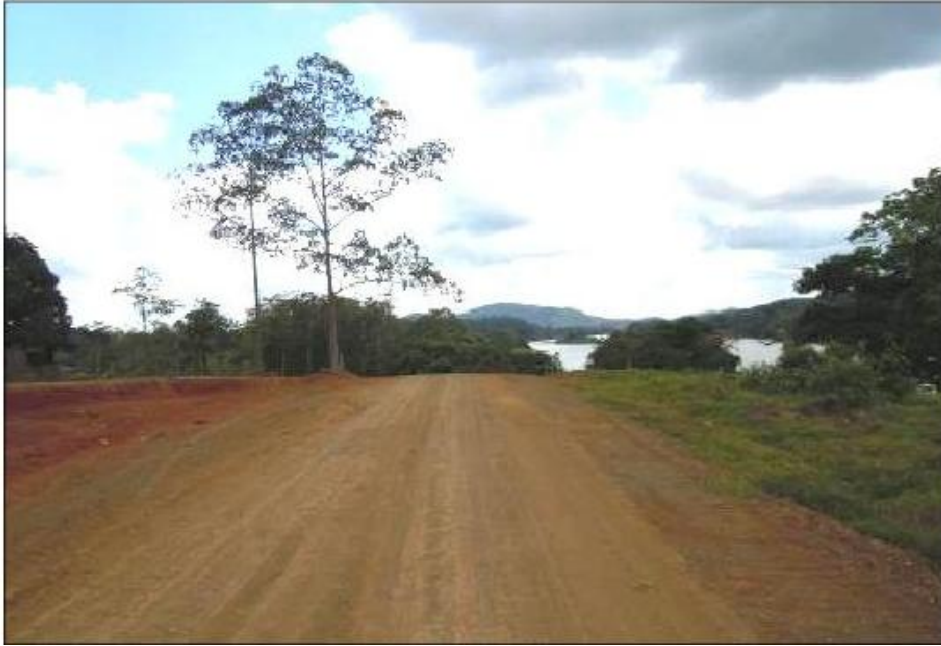
Figure 23. Subgrade level in road section 5. Source: LanammeUCR, May 2012
