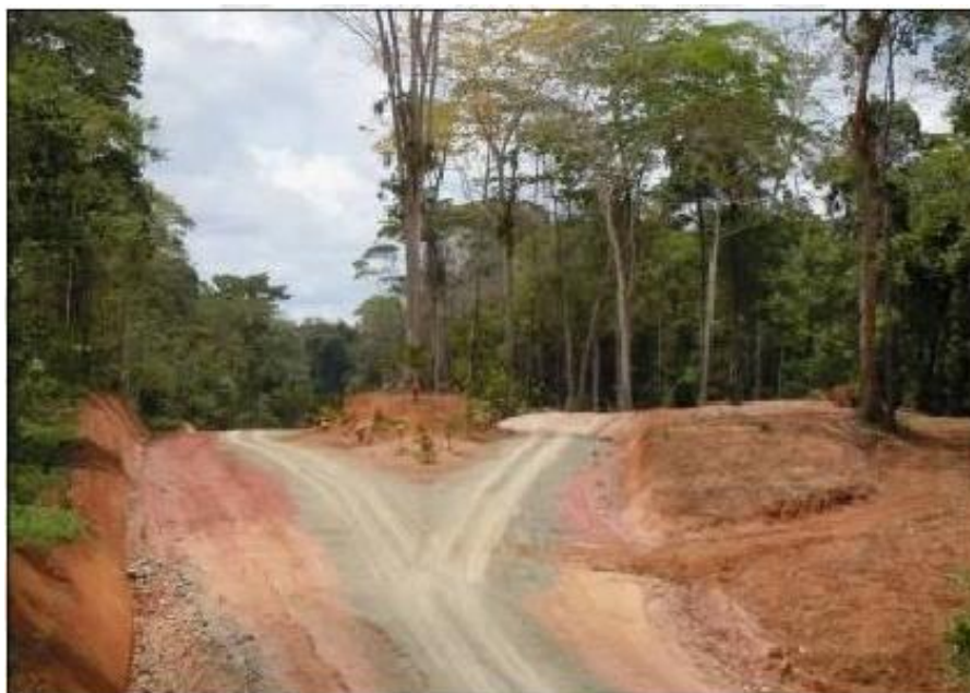
Figure 43. Road section bypassing existing trees, road section 8. Source: LannameUCR, May 2012
