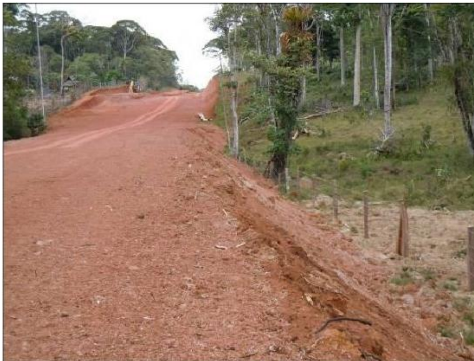
Figure 47. Fill areas without drainage structures. Source: LanammeUCR, May 2012
