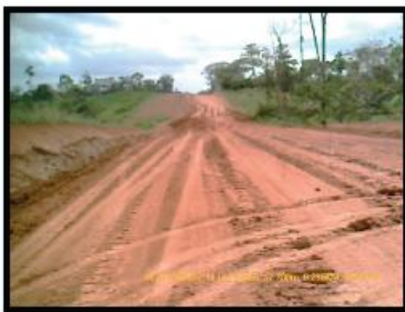
F44. View of a dirt stretch.
