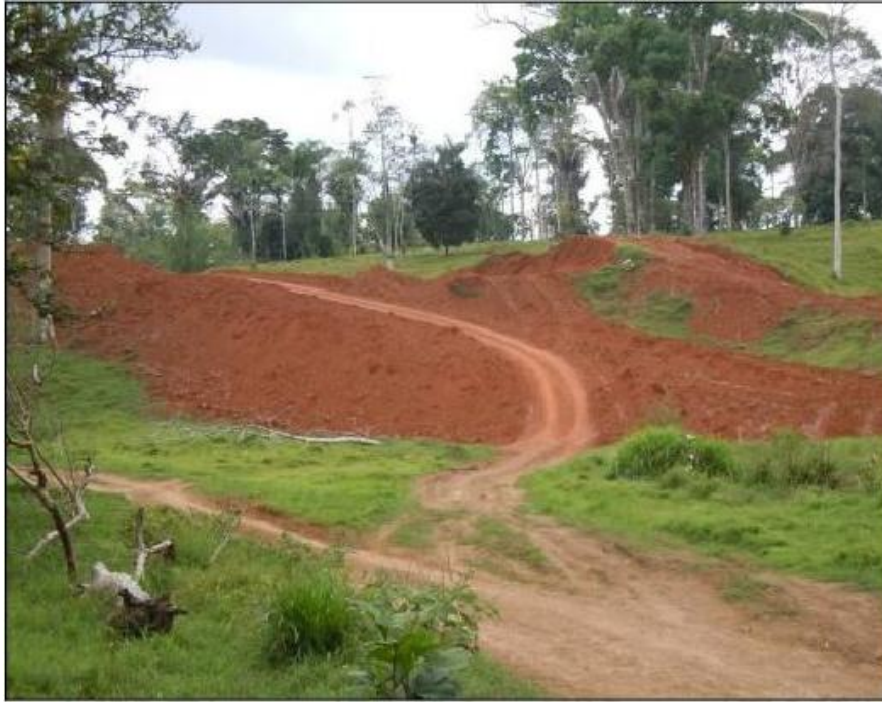
Figure 19. Fills found in road section 4.
