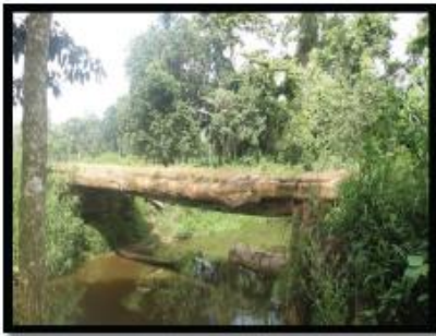
F13. Different bridges on wooden pillars can be observed.
