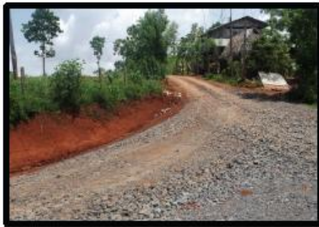
F38. Dirt road from Route 760 El Parque.
