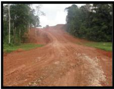
F14. A dirt road with no drainage; as it was not based on plans, disorganized cuts and fills were carried out.
