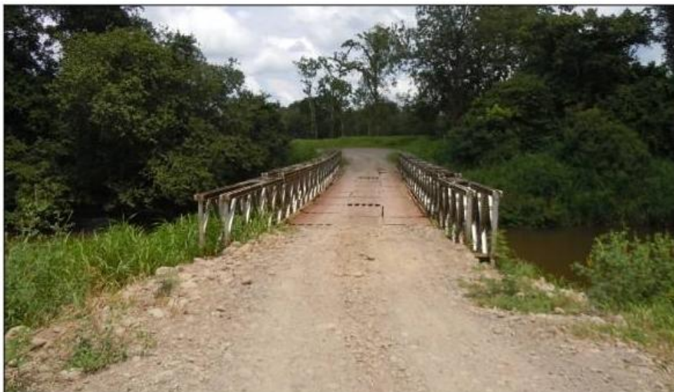
Figure 5. Bailey bridge on Fátima-Sarapiquí River Mouth road section. Source: LannameUCR, May 2012
