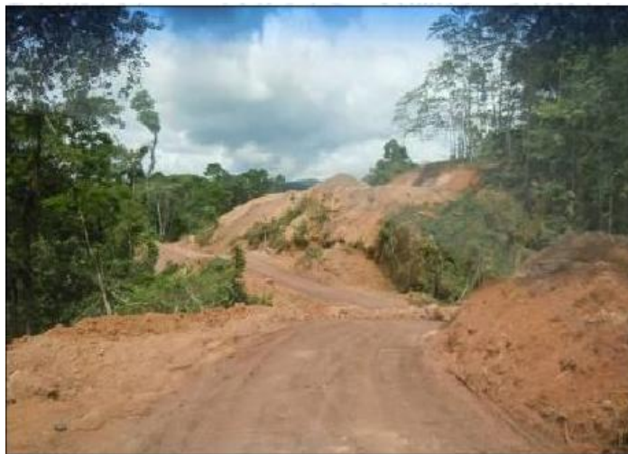
Figure 26. Cut and fill area, road section 6. Source: LanammeUCR, May 2012
