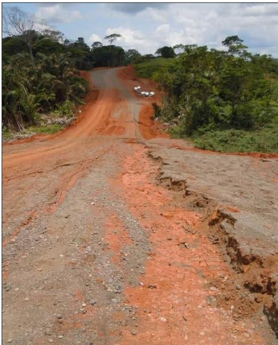
Figure 20. Sand laid over the subgrade in road section 4. Source: LanammeUCR, May 2012
