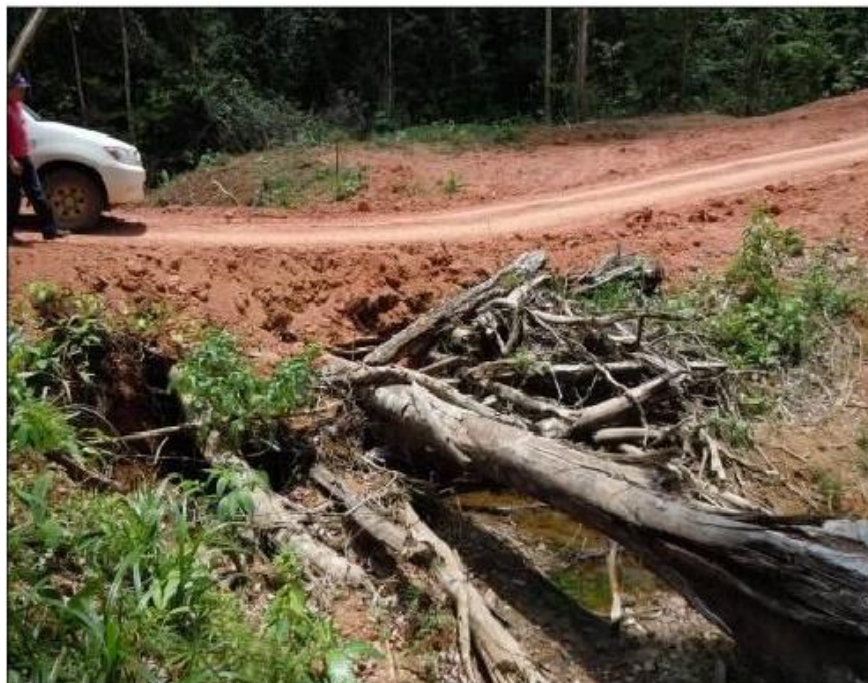
Figure 40. Provisional log stream crossing, road section 8. Source: LannameUCR, May 2012
