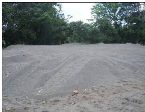
Figure 24. Subgrade level in road section 5. Source: LannameUCR, May 2012
