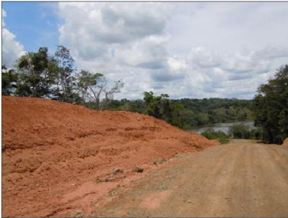
Figure 39. Excavated material mound, road section 8. Source: LannameUCR, May 2012
