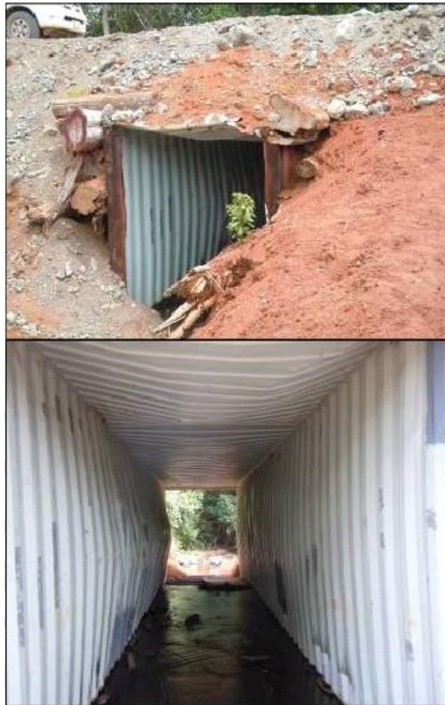
Figure 46. Containers used as square culvert pipes.
