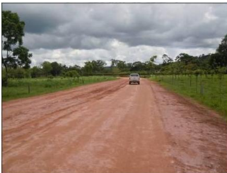
Figure 13. Fill section, road section 3. Source: LannameUCR, May 2012
