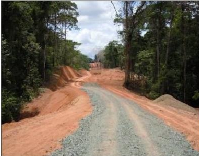
Figure 41. Beginning of area with granular material, road section 8. Source: LannameUCR, May 2012
