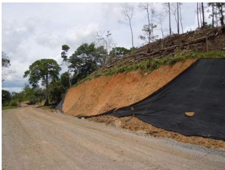
Figure 36. Scattered placing of woven material on slopes. Source: LannameUCR, May 2012
