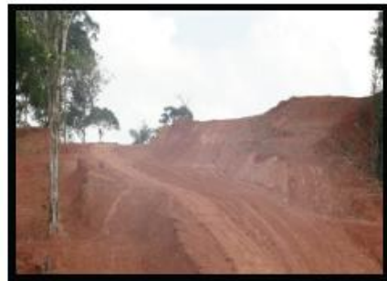
F14. A dirt road with no drainage; as it was not based on plans, disorganized cuts and fills were carried out.
