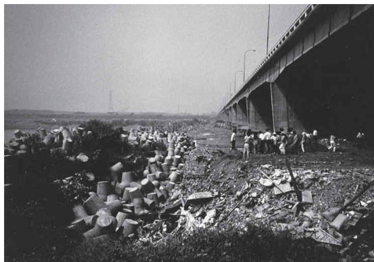
Figure 13. Undercutting and grade control efforts along the downstream side of the Kaoping Bridge over the Kaoping River, Taiwan, to control incision caused by massive gravel mining downstream. (Photograph by the author, October 1995.)
