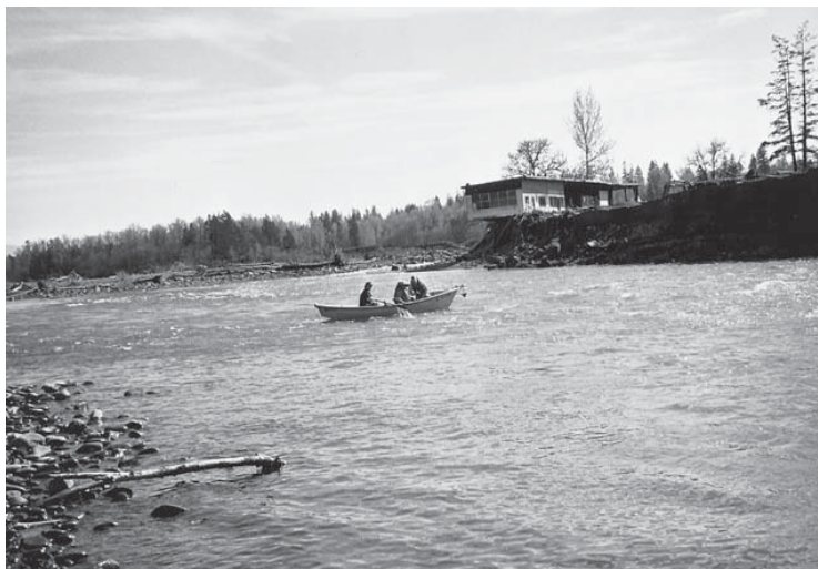
Figure 17. Building undercut by bank erosion as the Clackamas River flows through a captured gravel pit near Barton, Oregon. (Photograph by the author, April 1996.)
