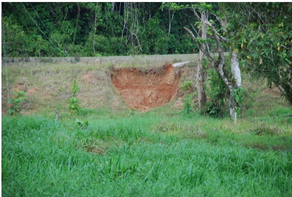
Figure 3.4. May 2014 photograph of erosion resulting from direct drainage from road onto fill.
