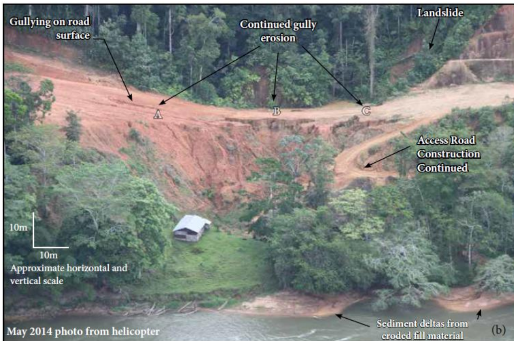
Figure 2.11. Severely Eroding Site 9.6, 18.2 km downstream of Mojon II. Oblique aerial view from May 2014.
