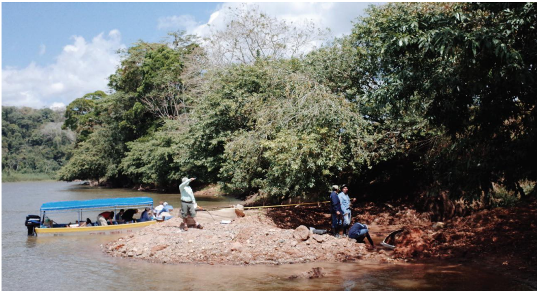
Figure 2.24. Delta deposit from fill material of failed crossing 20.3 km downstream of Mojon 2 extending into the San Juan River. Photograph from March 31, 2014.
