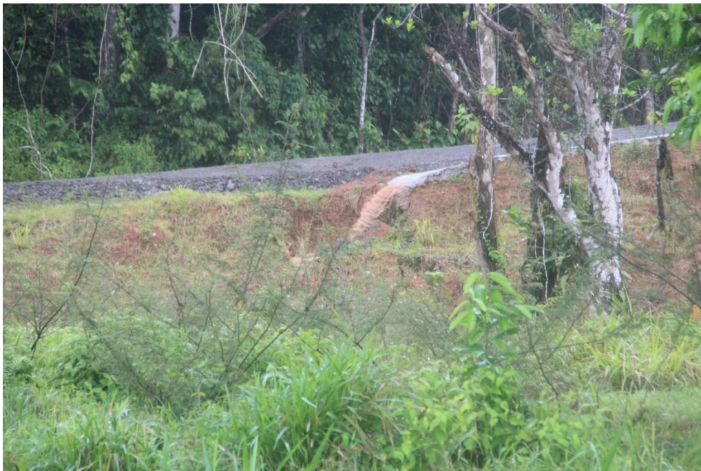
Figure 3.4. May 2014 photograph of erosion resulting from direct drainage from road onto fill.
