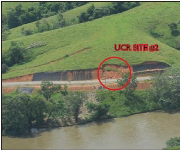
Figure 2.35. Aerial image of UCR Site 2: Landslide on cut slope.
