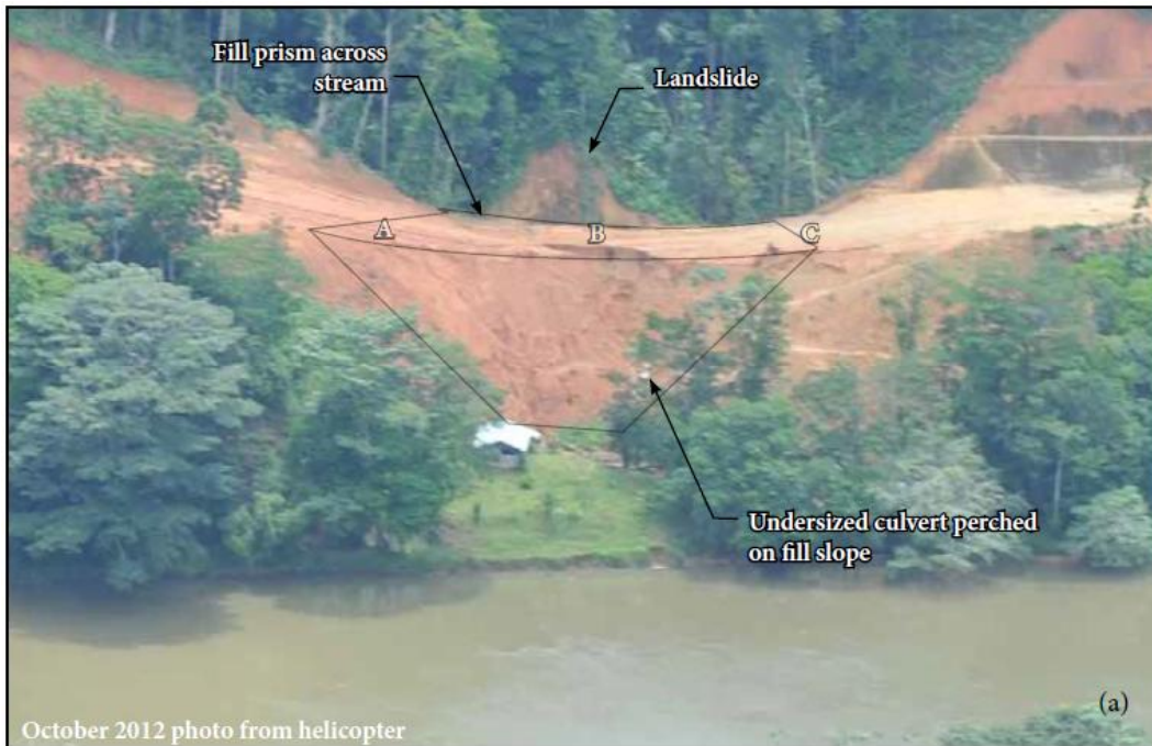
Figure 2.9. Severely Eroding Site 9.6, 18.2 km downstream of Mojon II. Oblique aerial view from October 2012.
