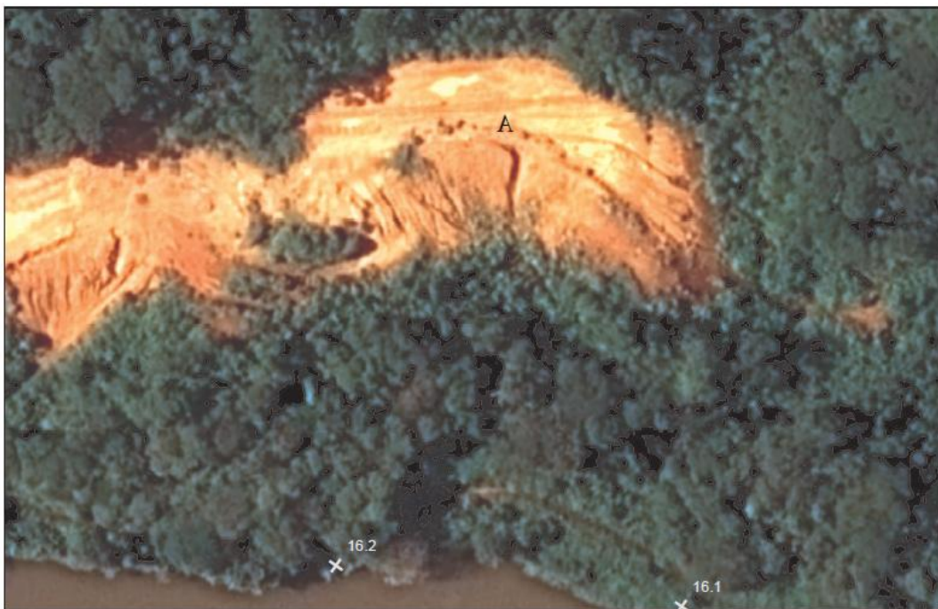
Figure 2.16. Severely Eroding Site 8.1, 16.1 km downstream of Mojon II. High-resolution satellite image of December 2013.
