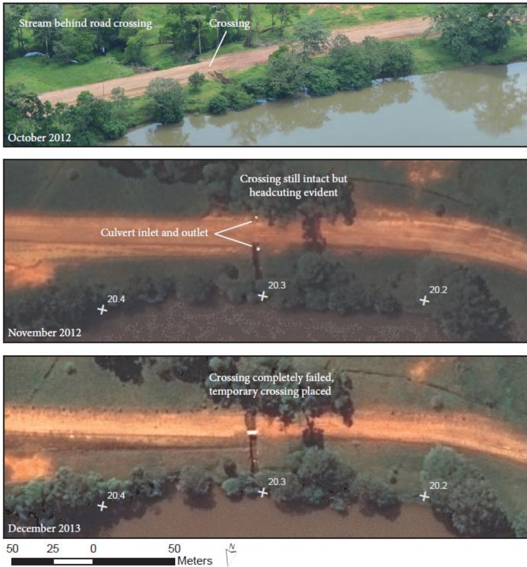
Figure 2.12. Helicopter and satellite imagery of failed fill crossing on flat land 20.3 km downstream of Mojon II.
