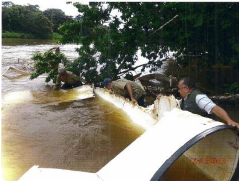
Figure 2.5. Removal of culvert fragments from San Juan River adjacent to Severely Eroding Site 9.4, 18.0 km downstream of Mojon II. Photograph from October 27, 2013.
