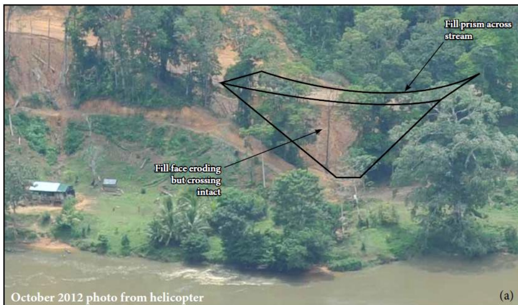
Figure 2.2. Severely Eroding Site 9.4, 18 km downstream of Mojon II. Oblique aerial view from October 2012.
