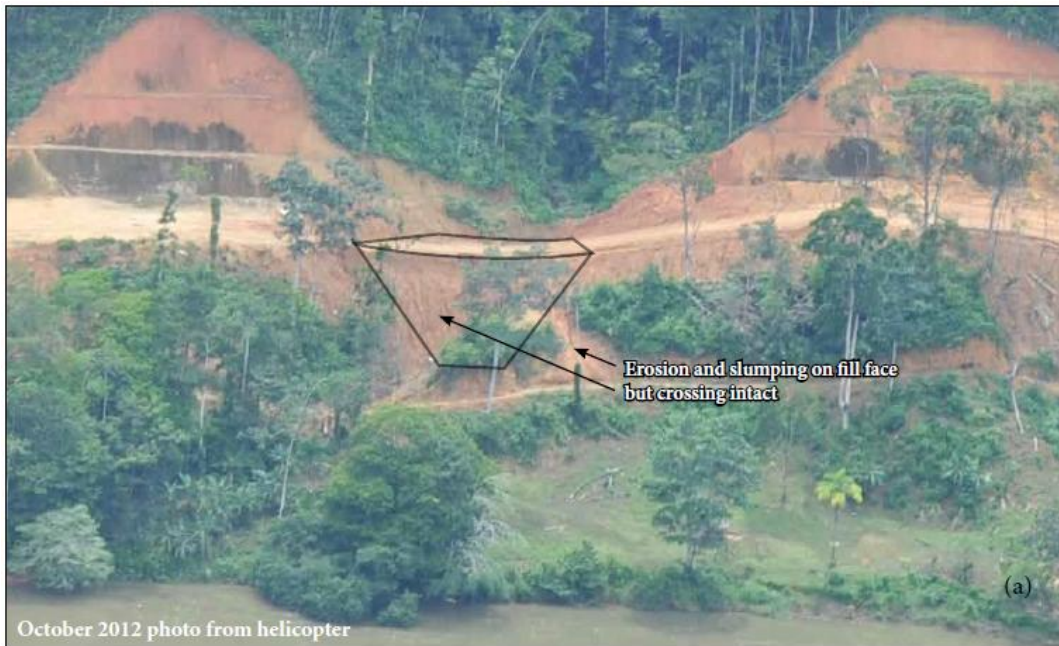
Figure 2.6. Severely Eroding Site 9.5, 18.1 km downstream of Mojon II. Oblique aerial view from October 2012.
