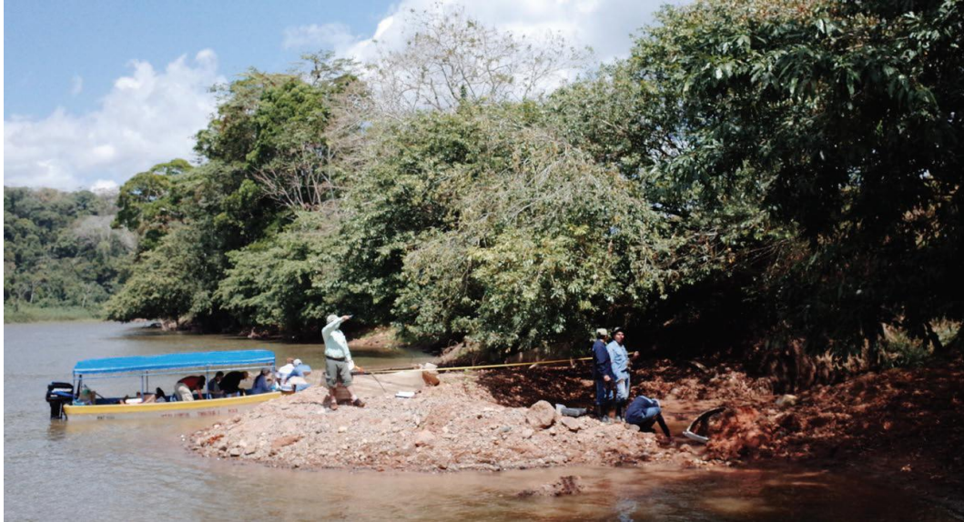
Figure 5.4. Delta deposit from fill material of failed crossing 20.3 km downstream of Mojon 2 extending into the San Juan River. Photograph from March 31, 2014.
