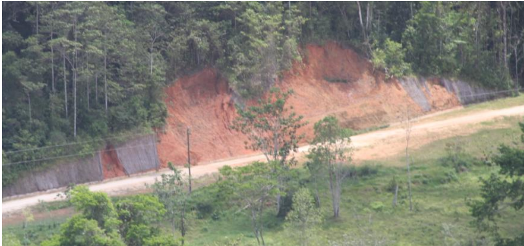
Figure 3.1. Failing geotextile approximately 10.0 km downstream from Mojon II.
