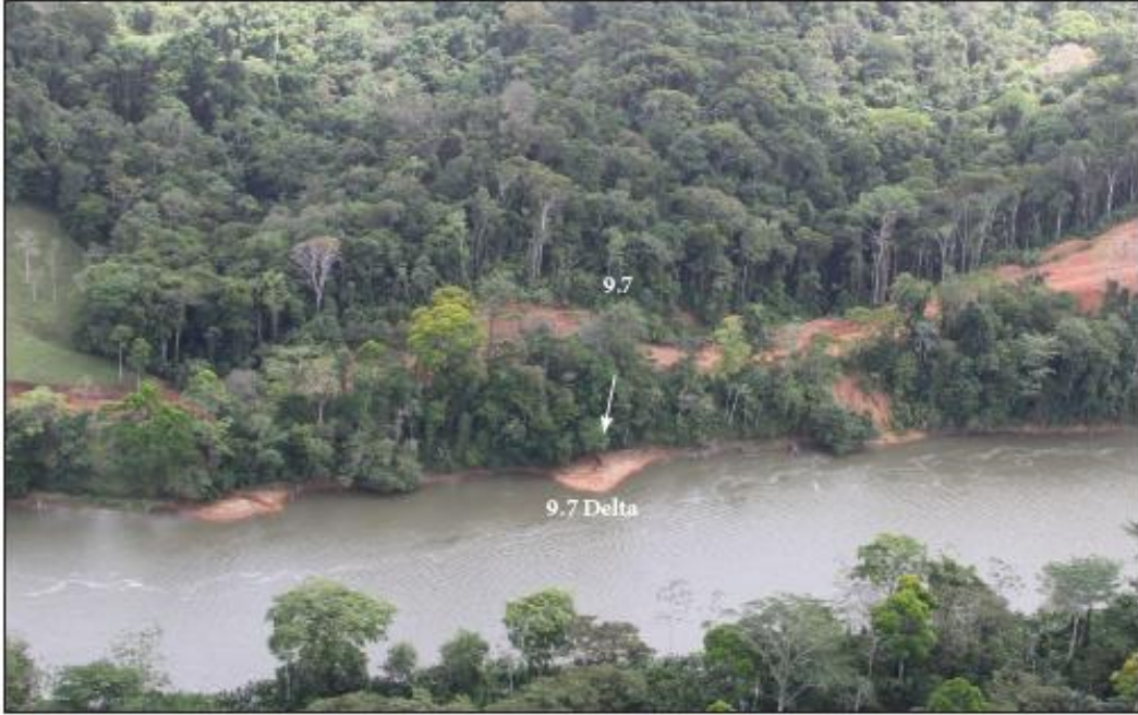
Figure 2.25. Delta deposit from Severely Eroding Site 9.7. Aerial photograph from May 2, 2014.
