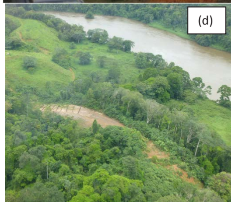
Figure 7.16 Path cleared for the Road near Crucitas, just east of the Río Infiernito (a) on 15 February when unmanaged runoff from the path cleared in preparation for construction of the road bed had caused sheet and rill erosion (b) The same area on 7 May 2013 after installation integrated measures to manage runoff involving regrading, silt fences, and concrete-lined outboard ditch (c) in April 2014, nothing had changed significantly and in August 2014 it was apparent that erosion mitigation continued to be successful and that no sediment from the site was reaching the Río San Juan. Photographs by author.
