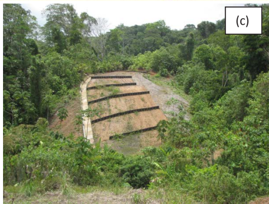
Figure 7.16 Path cleared for the Road near Crucitas, just east of the Río Infiernito (a) on 15 February when unmanaged runoff from the path cleared in preparation for construction of the road bed had caused sheet and rill erosion (b) The same area on 7 May 2013 after installation integrated measures to manage runoff involving regrading, silt fences, and concrete-lined outboard ditch (c) in April 2014, nothing had changed significantly and in August 2014 it was apparent that erosion mitigation continued to be successful and that no sediment from the site was reaching the Río San Juan. Photographs by author.
