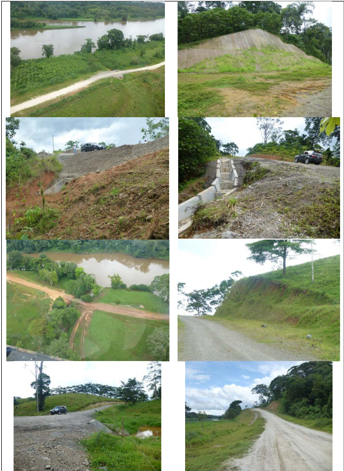
Figure 7.7 Condition of additional CONAVI erosion mitigation works inspected by the author in 2014: left watercourse crossings, and right slopes. Photographs by author.
