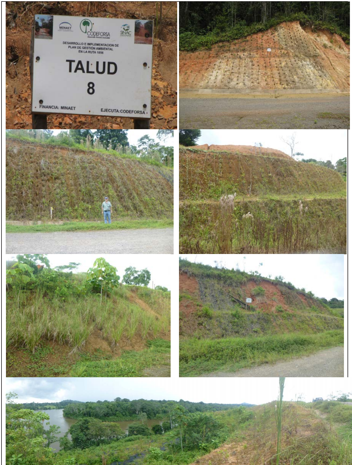
Figure 7.6 Condition of some of the slopes revegetated by CODEFORSA that were visited in 2014. Photographs by the author.
