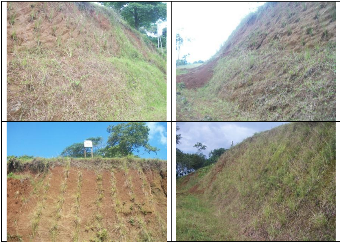
Figure 7.2 Slope 9 (near Tiricias) in February 2014, following treatment by CODEFORSA for surface protection (example taken from 2014 CODEFORSA Report)
