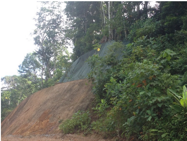
Photo 4: Sedimentation mitigation measures in section Infiernito river-Boca San Carlos.
