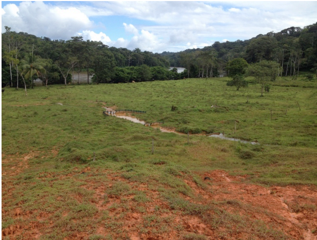
Photo 3: Sedimentation mitigation measures in section Infiernito river-Boca San Carlos.
