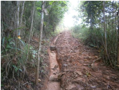
Drain on terrace, Slope T75
