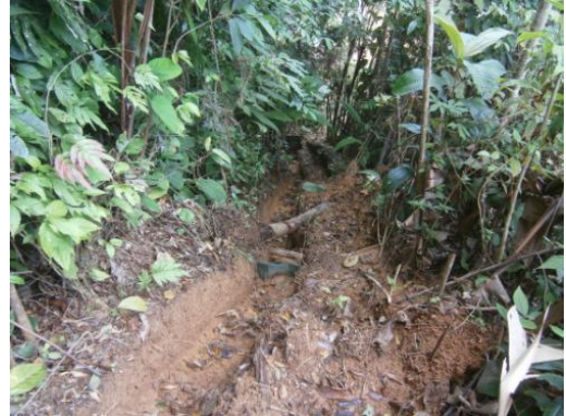
Upper drain, Slope T73a.
