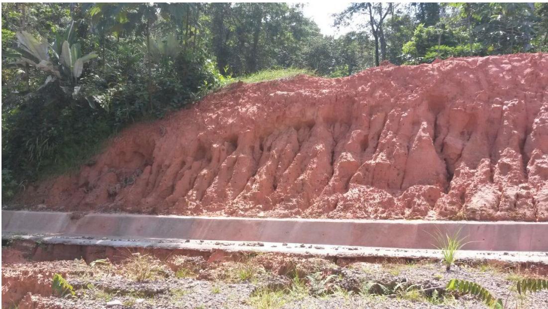
Figure 21. Photograph of Site 10 on October 22, 2014.
