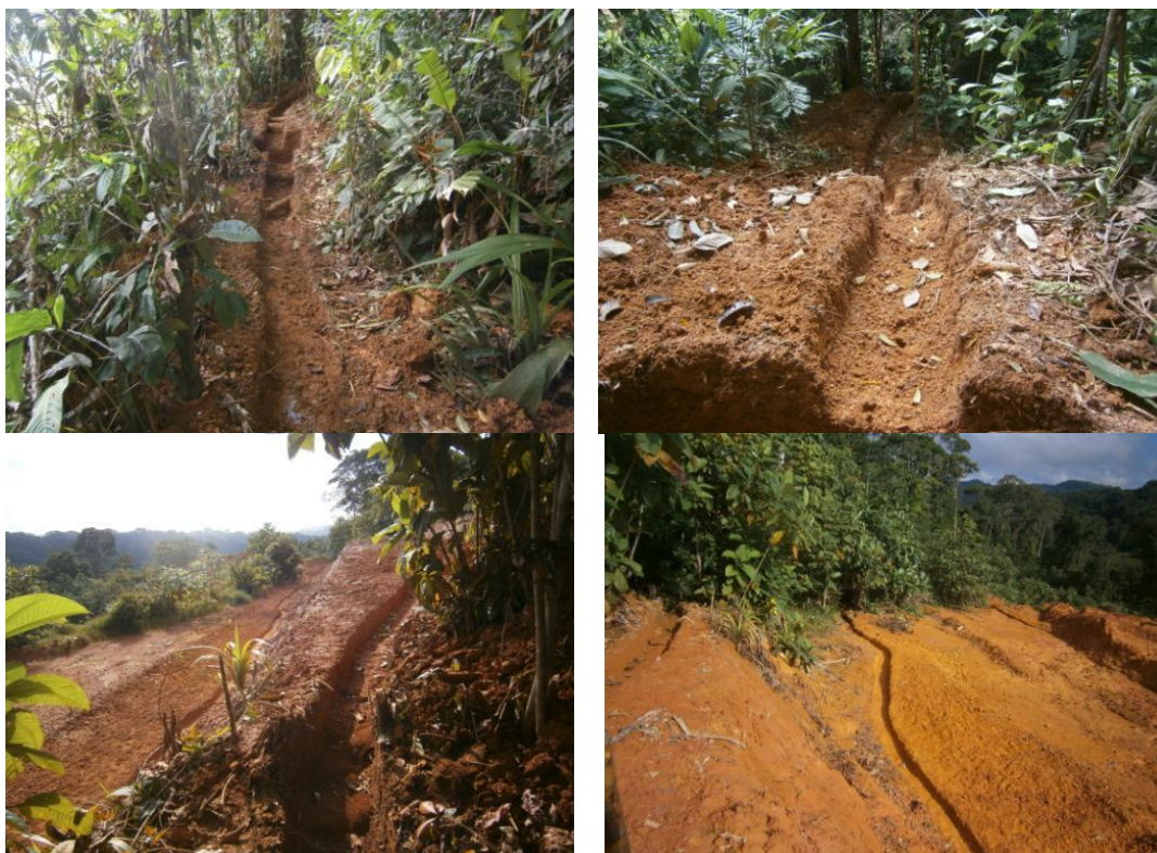
Construction of drain in the terraces.
