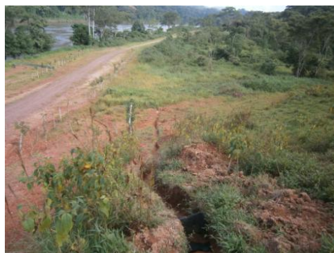
Drain on upper part of cut, Slope T82a.
