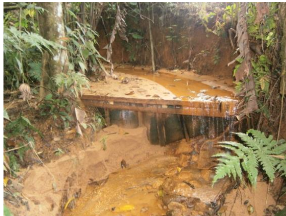
Sediment trap functioning, downstream between slopes T69 and T71.
