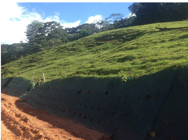
Photo 6: Slope contention in section Infiernito river-Boca San Carlos.
