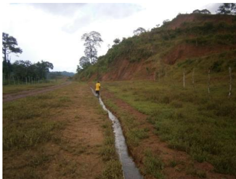
Drain at base of cut, Slope T81.
