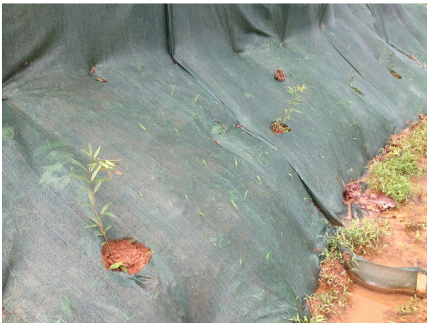
Photo 10: Sotacaballo trees planted on saran-covered slopes in Chorreras sector
