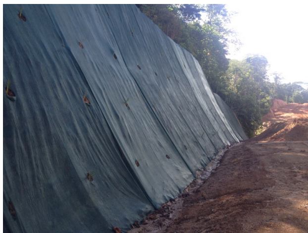
Photo 7: Slope contention in section Infiernito river-Boca San Carlos.
