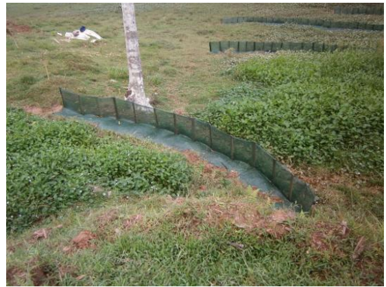
Construction of sediment traps downstream from the creek at the end of slope T76 b.
