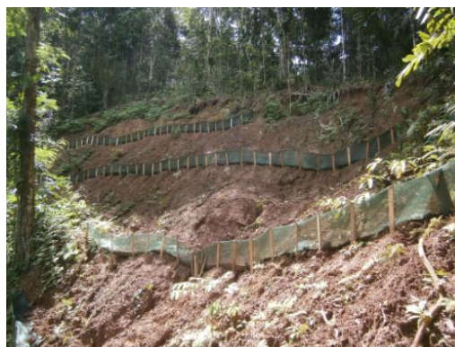
Large sediment trap, Slope T66a.
