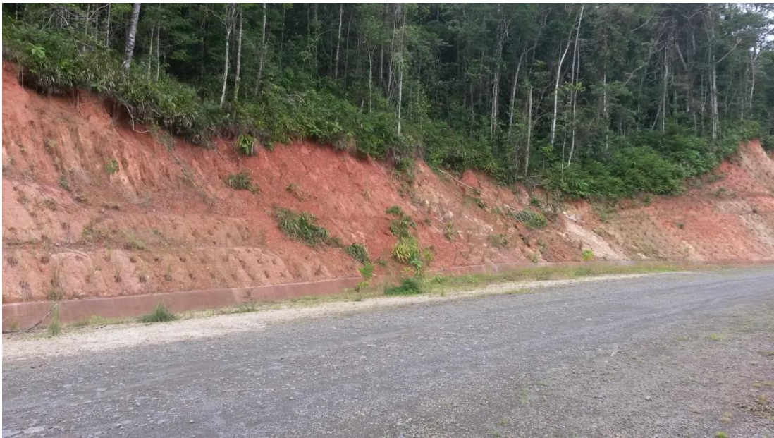
Figure 12. Cut slope adjacent to Site 4 on August 19, 2014.
