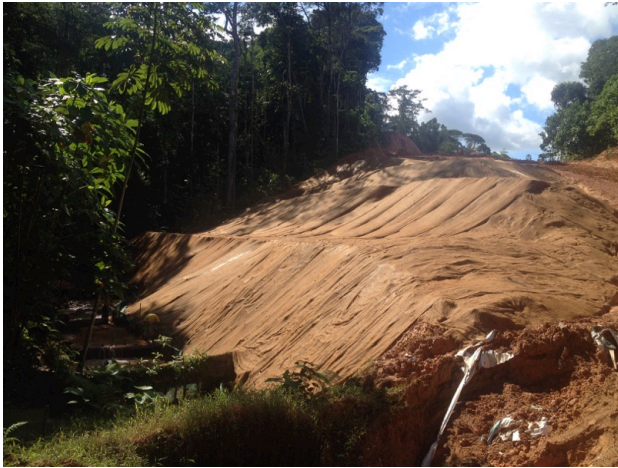
Photo 8: Slope contention in section Infiernito river-Boca San Carlos.
