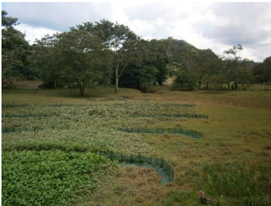
Construction of sediment traps downstream from the creek at the end of slope T76 b.
