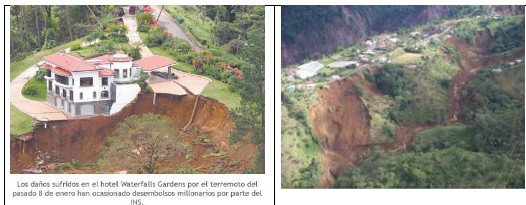
Fig. 10. Photographs of landslides triggered in January 2009 showing the types of damage caused by the Cinchona earthquake (see Figure 9 for location).
