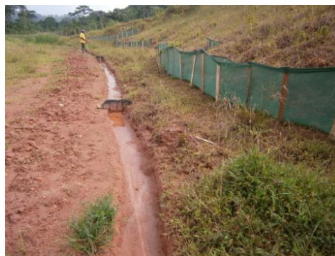
Drain at base of filling, Slope T82b.
