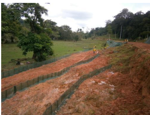
Large sediment trap, Slope T76b.
