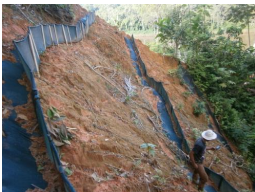
Large sediment trap, Slope T69a.
