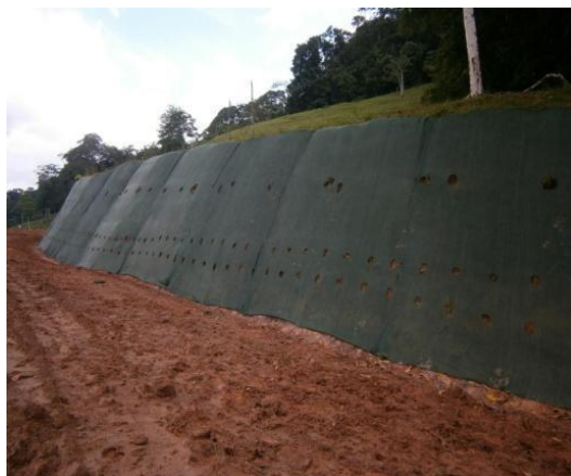
Placement of saran on Slope T76a.
