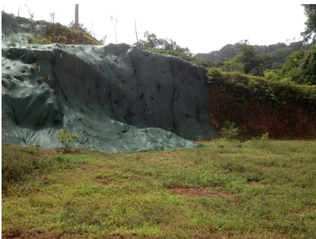
Photo 11: Sedimentation mitigation measures in the Chorreras sector.
