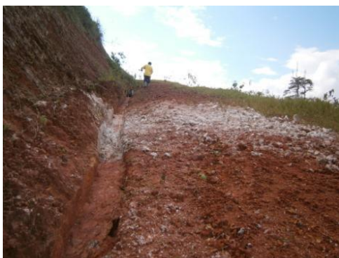
Drain on terrace, Slope T81
