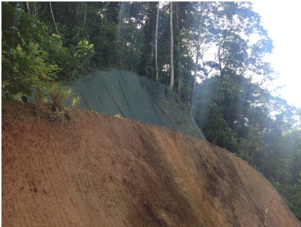
Photo 9: Slope contention in section Infiernito river-Boca San Carlos.
