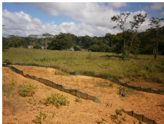
Large sediment trap, Slope T66b.
