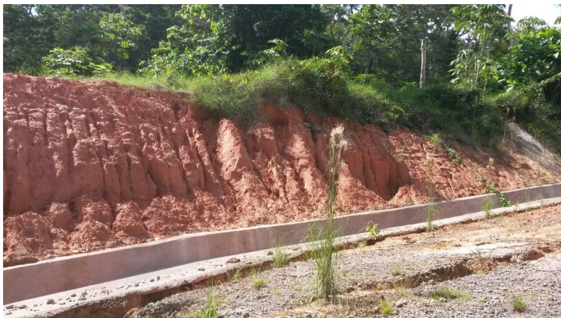
Figure 22. Photograph of Site 10 on October 22, 2014.
