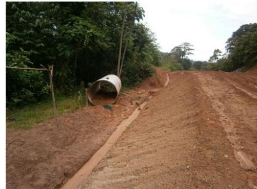
Drain on road, Slope T75.
