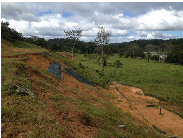
Photo 5: Sedimentation mitigation measures in section Infiernito river-Boca San Carlos.
