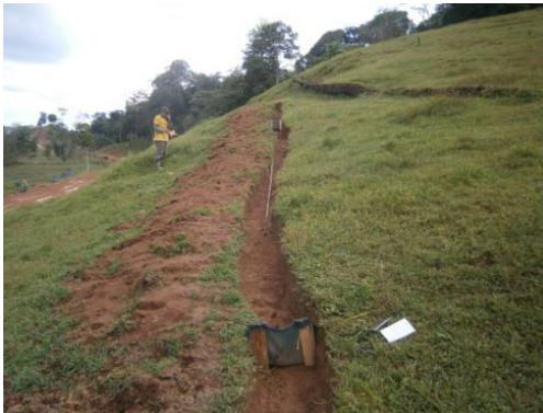
Upper drain, Slope T66a.
