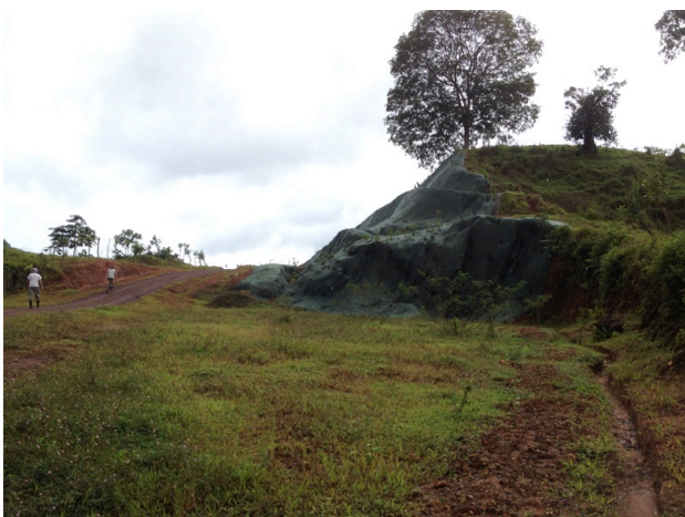
Photo 12: Sedimentation mitigation measures in the Chorreras sector.
