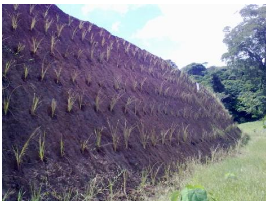
View of Slope No. 10
