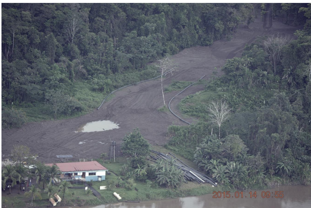
Photograph 2: Sediment deposit site north of Nicaraguan Delta army post Coordinates 10°46'26.44"N 83°45'55.09"O
