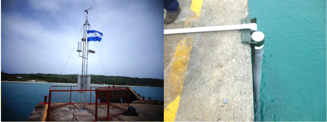
Corn Island Tide Gauge Station installed in June 2014
