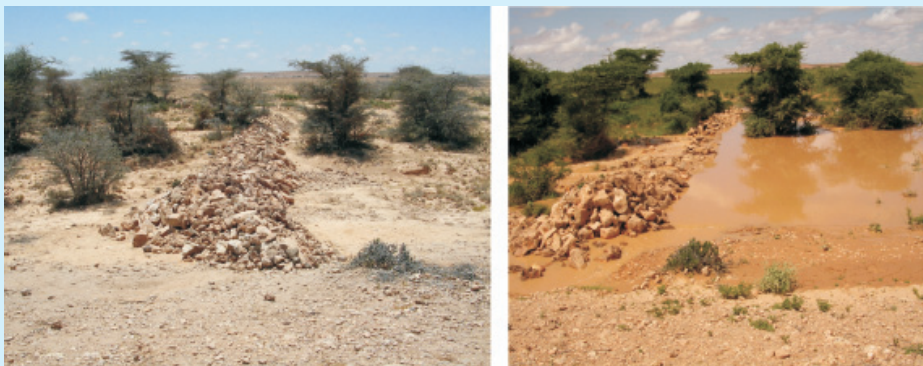
Simple rock dam at Awsane built in March 2005 (left) before the rains and two months later after rain (right)
