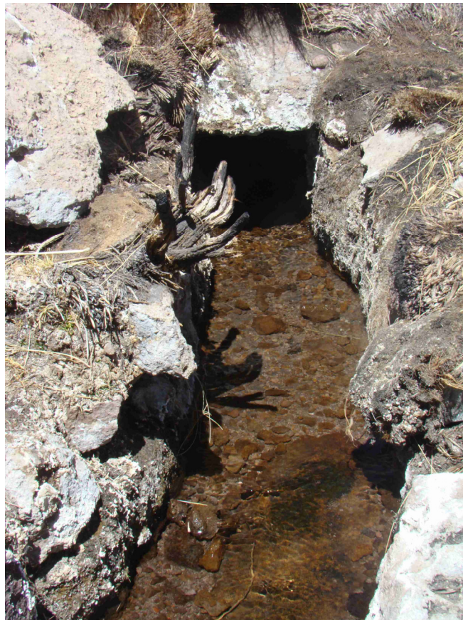
Figure 17: Silala spring directly connected to an artificial channel where the spring emerges from the formation (Source: DIREMAR, 2016)
