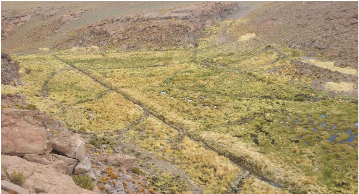
Figure 15: The extensive network of artificial drainage mechanisms crossing the bofedales in the North (Cajones) Ravine of the Silala in Bolivia (Source: DIREMAR, 2017)
