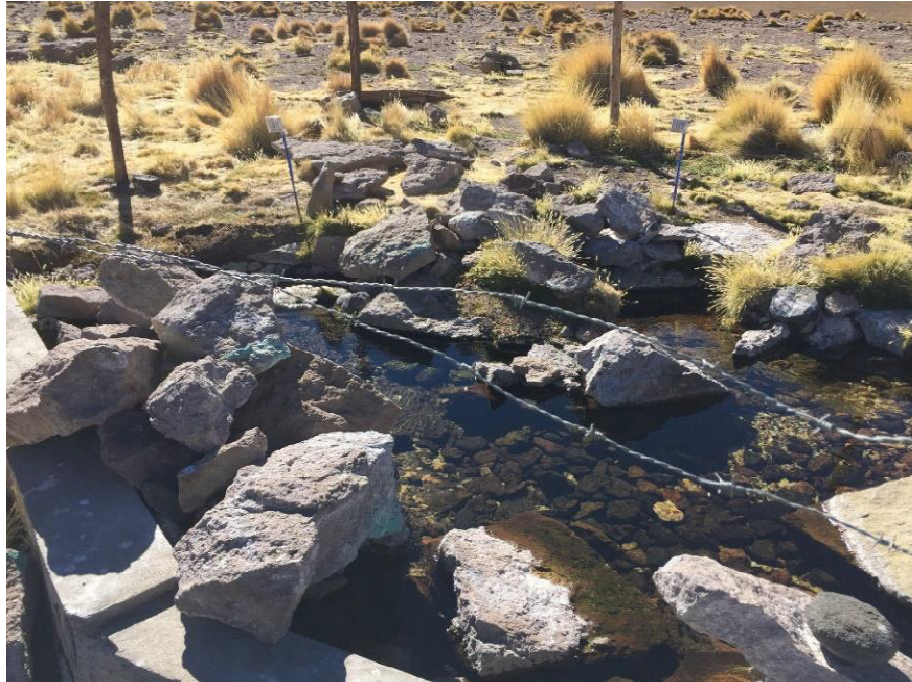
Figure 19: Rocks adjacent to channels and drainage mechanisms providing evidence of explosive blasts used to lower spring elevations and increase spring discharge (Source: Annex F, in DHI, Final Report, p. 97)
