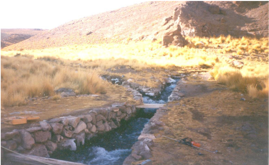
Figure 8: The technical stonework of the Main Channel as it receives water transported by the two main subsidiary channels emerging from the North (Cajones) Ravine and South (Orientales) Ravine (Source: DIREMAR, 2018).
