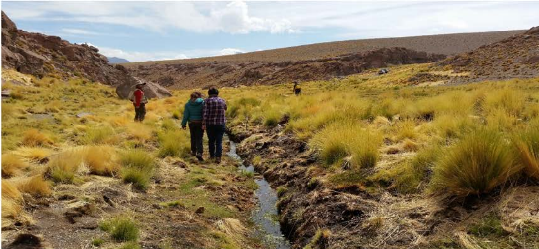
Figure 8 Northern wetland facing downstream. Exposed peat soil faces are visible along the canal.
