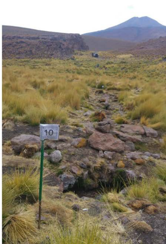
Figure 10 Photo showing exposed springs piped directly to the main canal.
