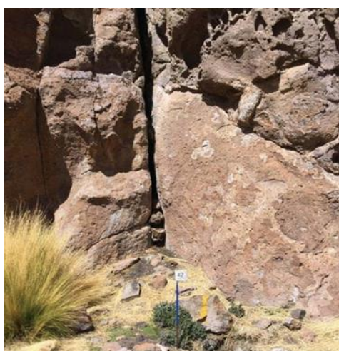
Figure 7-5 Example of fracturing in the ignimbrite that is coincident with spring discharge, and represents transmission of groundwater to the surface
