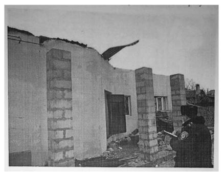
Photo No. 1: Damaged building located at number **17 Nezhynska Street:** no roof, charred walls, shattered window panes
