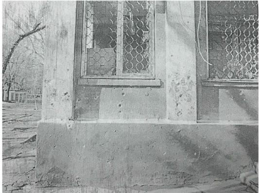
PHOTO No. 28: General view of damage to the building facade caused by falling shell fragments at the intersection of Lenin Street and Voznesenskoho Street, Kramatorsk, Donetsk Oblast (near 24 Lenin Street, in the backyard)
