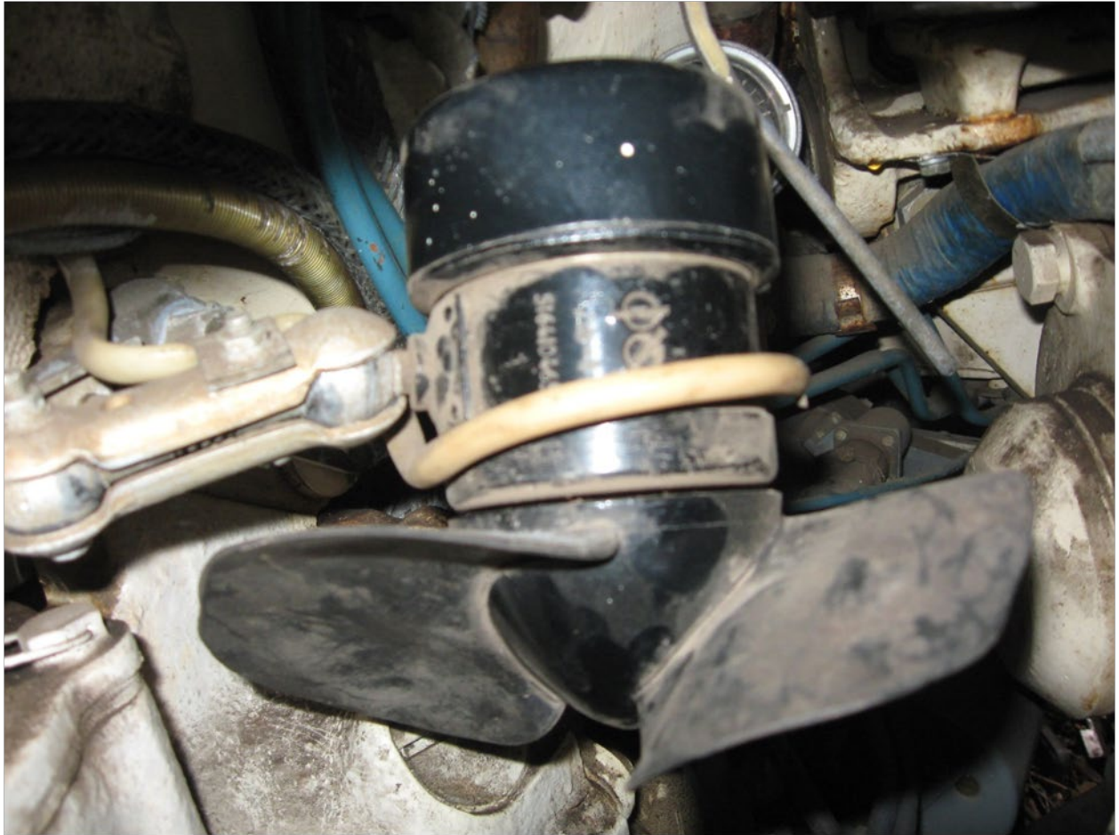
Fans of "ДВ-3" type at crew stations
