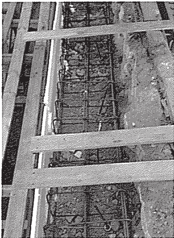
INSTALLATION OF REBARS
