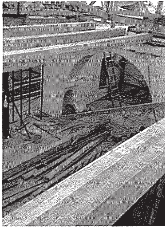
FULL DISMANTLING OF THE ROOF
