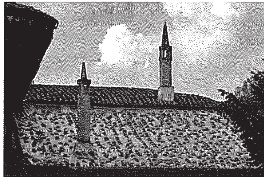
FRAGMENT OF ROOFING TILE, WHICH IS USED AS WEIGHTING FOR POLYETHYLENE COATING
