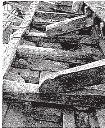
FRESH SAW - CUT OF THE AUTHENTIC BEAMS
