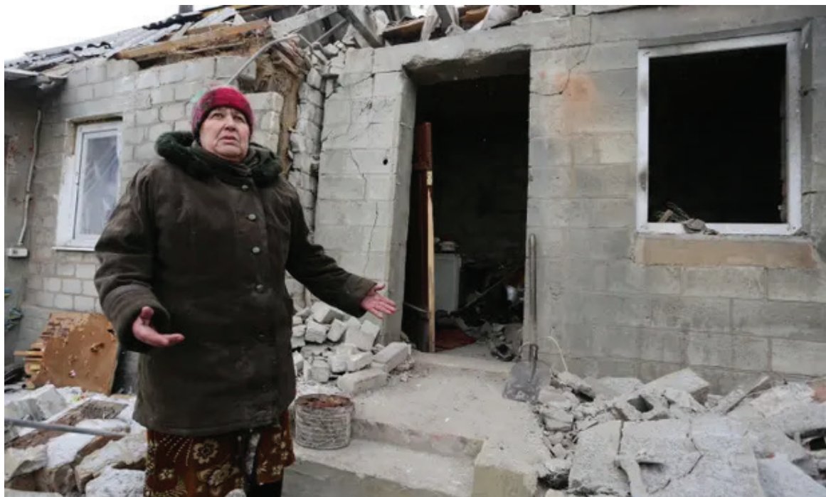
▲ Valentina, a 73-years-old resident of Avdiivka, stands outside her home damaged during the recent shelling. Photograph: Alexey Pavlovsky/AFP/Getty Images
