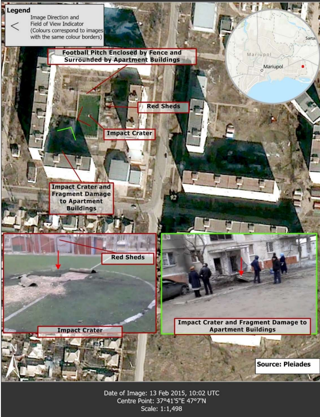
Figure 23. Mariupol Damage Graphic No. 5 (Open Source). 38
