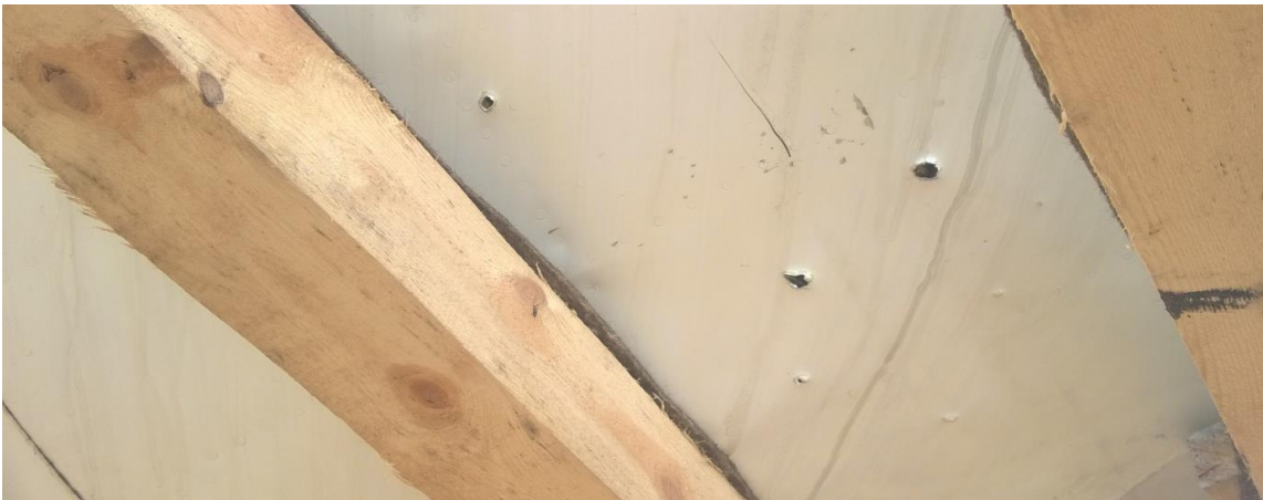
Figure 7.5 - Exit holes and non-penetrating damage to the starboard
