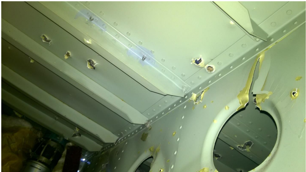
Figure 5.130 - Through-and-through holes in the cockpit floor (bottom view)
