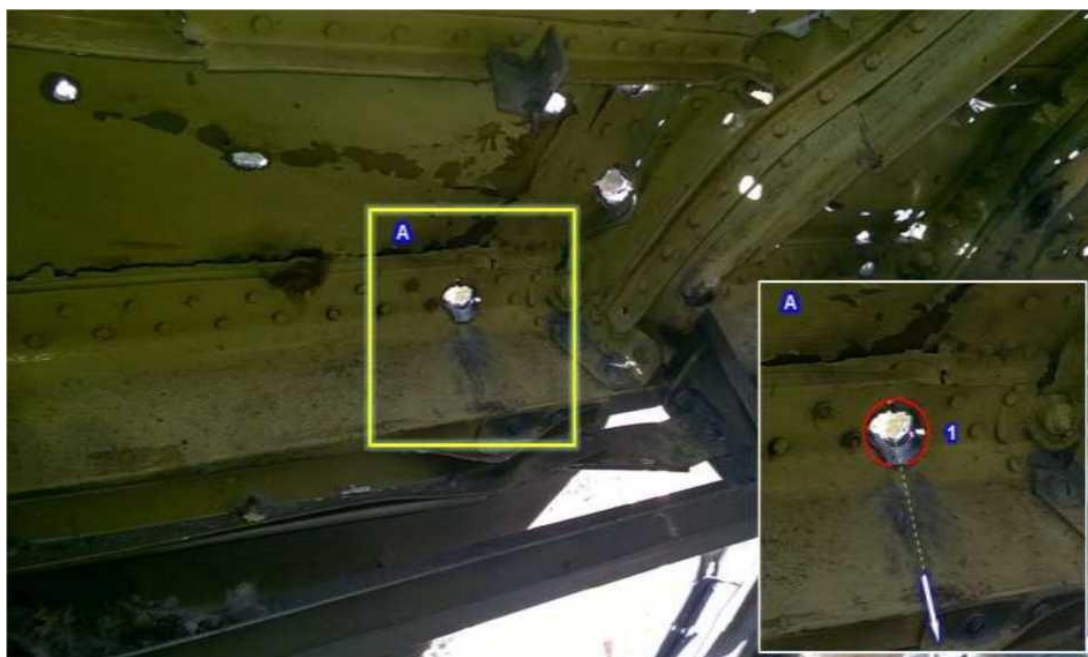
Figure A.4.13 - Direction of projectiles movement through the fragment of the upper port side (above the crew commander's window)
