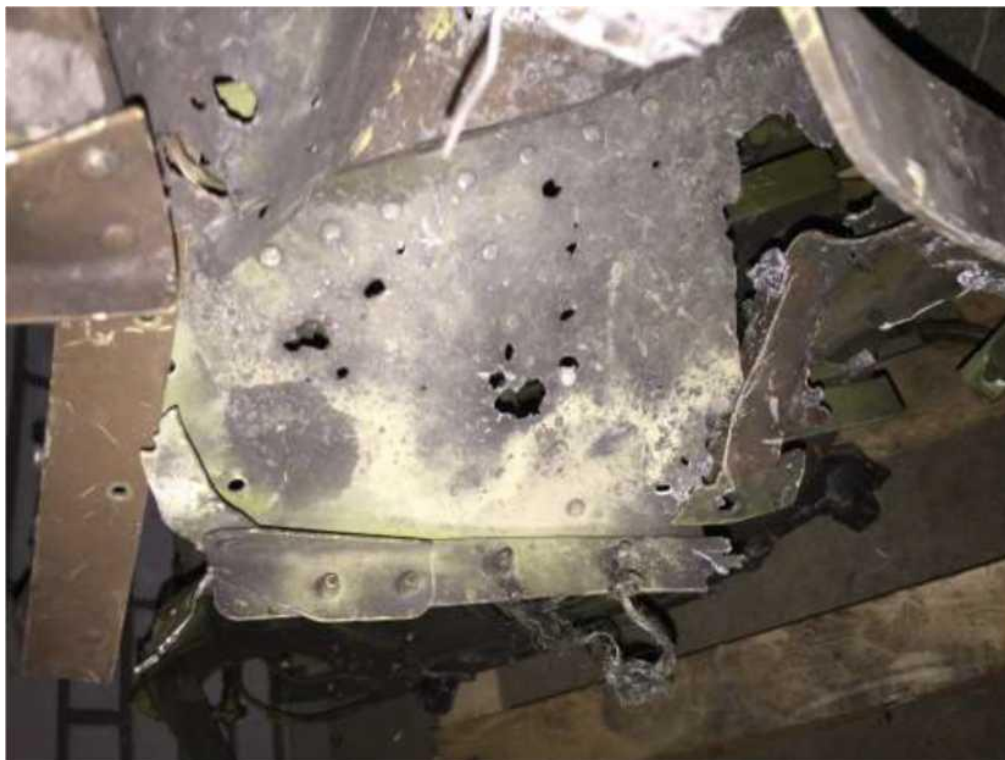
Figure 5.1.45 - Damage to cockpit floor and structural elements along the port side
