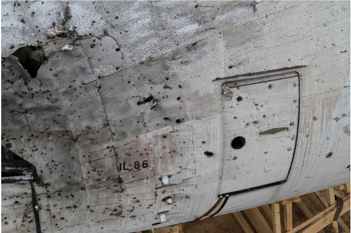
Figure 5.33 - Port side in L1 door area (overall view)
