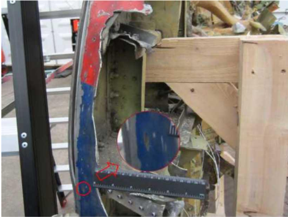
Figure 5.1.12 - Non-penetrating damage at the lower boundary of the coverage field in the area of the forward pressure bulkhead (STA 132.5). Approximate position of the coverage field boundary corresponds to the bottom cut of the measuring ruler
