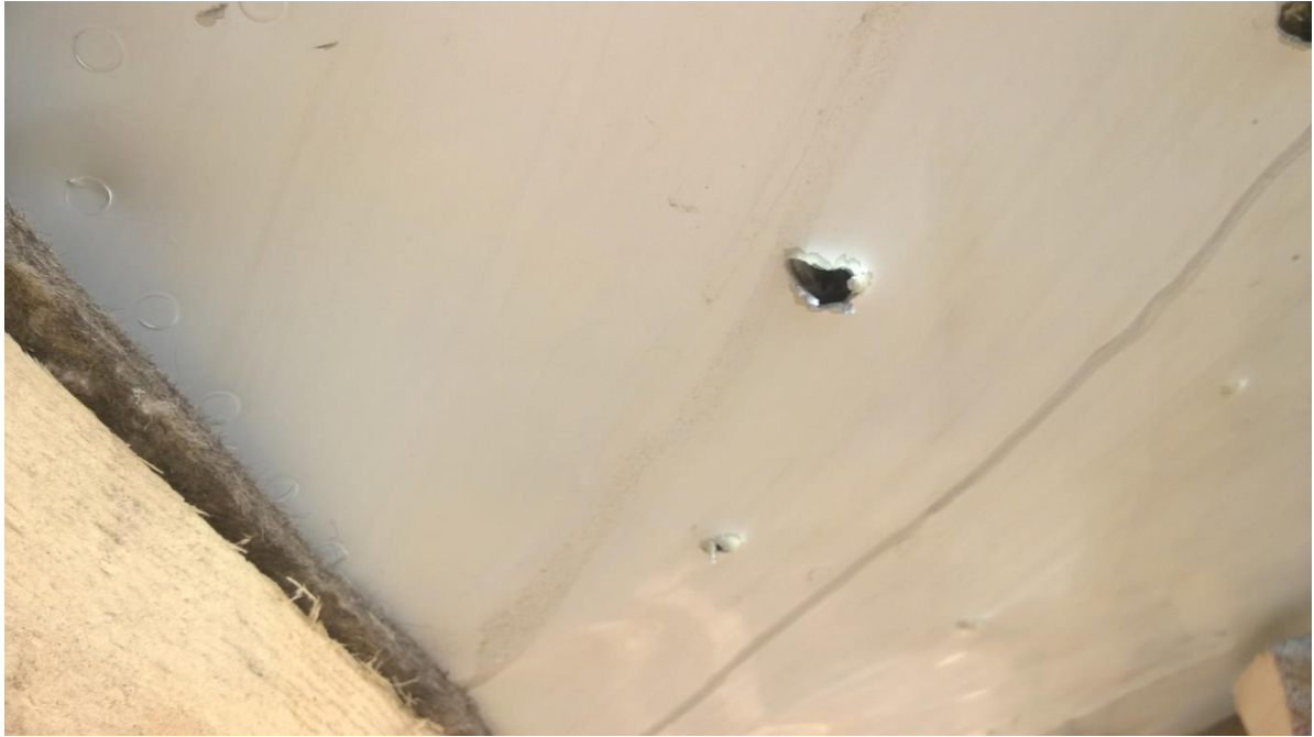
Figure 5.97 - Exit holes and non-penetrating damage
