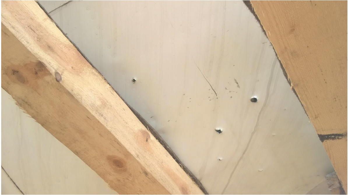
Figure 5.99 - Exit holes and non-penetrating damage
