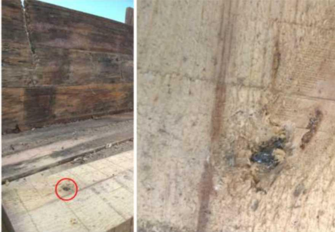
Figure 5.2.26 - Removing a ready-made impactor from the "L. 1" trap: left - depth of penetration of a ready-made impactor into the trap; right - ready-made impactor 9H314M 1-9 stuck in the trap
