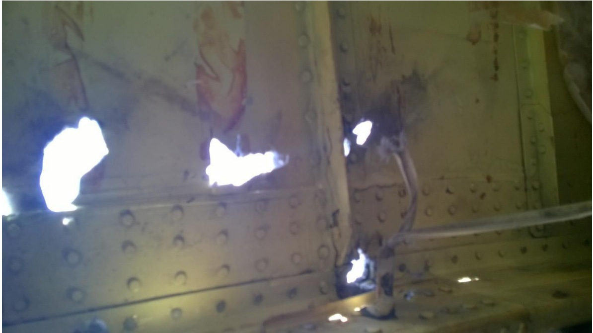
Figure 5.73 - Through-and-through holes in the cockpit roof (inside view)
