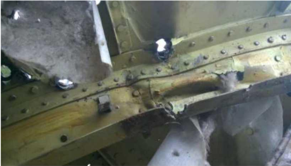
Figure B.3.20 - Characteristic view of the damage to the dovetails on the left side of the cockpit of the B-86 target aircraft (L-shaped reinforcements of the dovetails have been holed). The direction of motion of the projectiles is transverse to the structure of the aircraft. No piercing holes in the bulkheads
