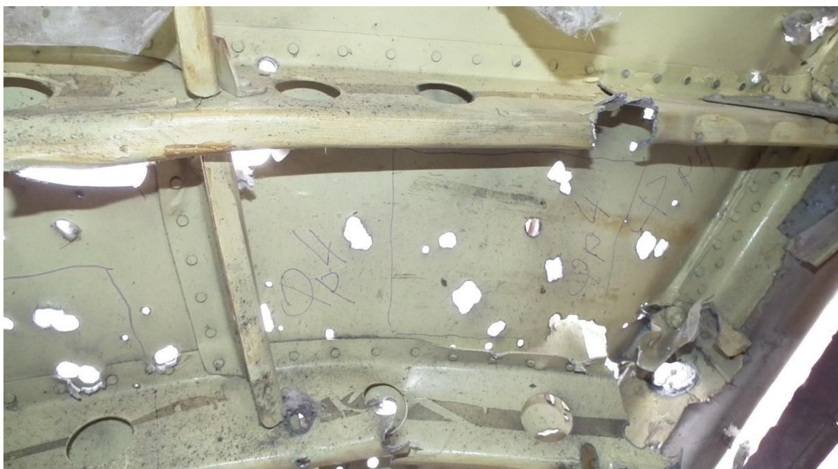
Figure 5.166 - Fragment No. 4 before extraction (internal view)
