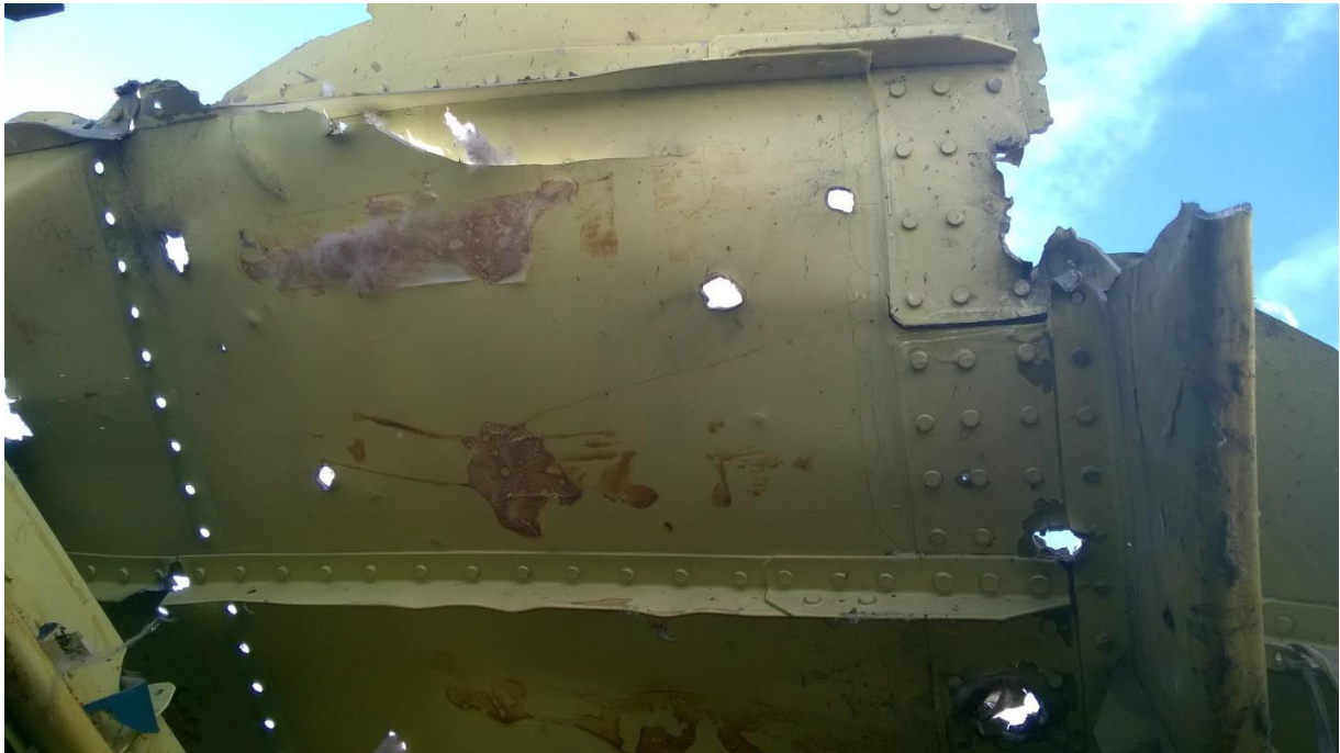
Figure 5.150 – Destruction of a frame (top of the port side)
