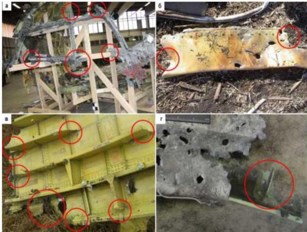
Figure 5.1.70 - Deformation and destruction of structural elements
