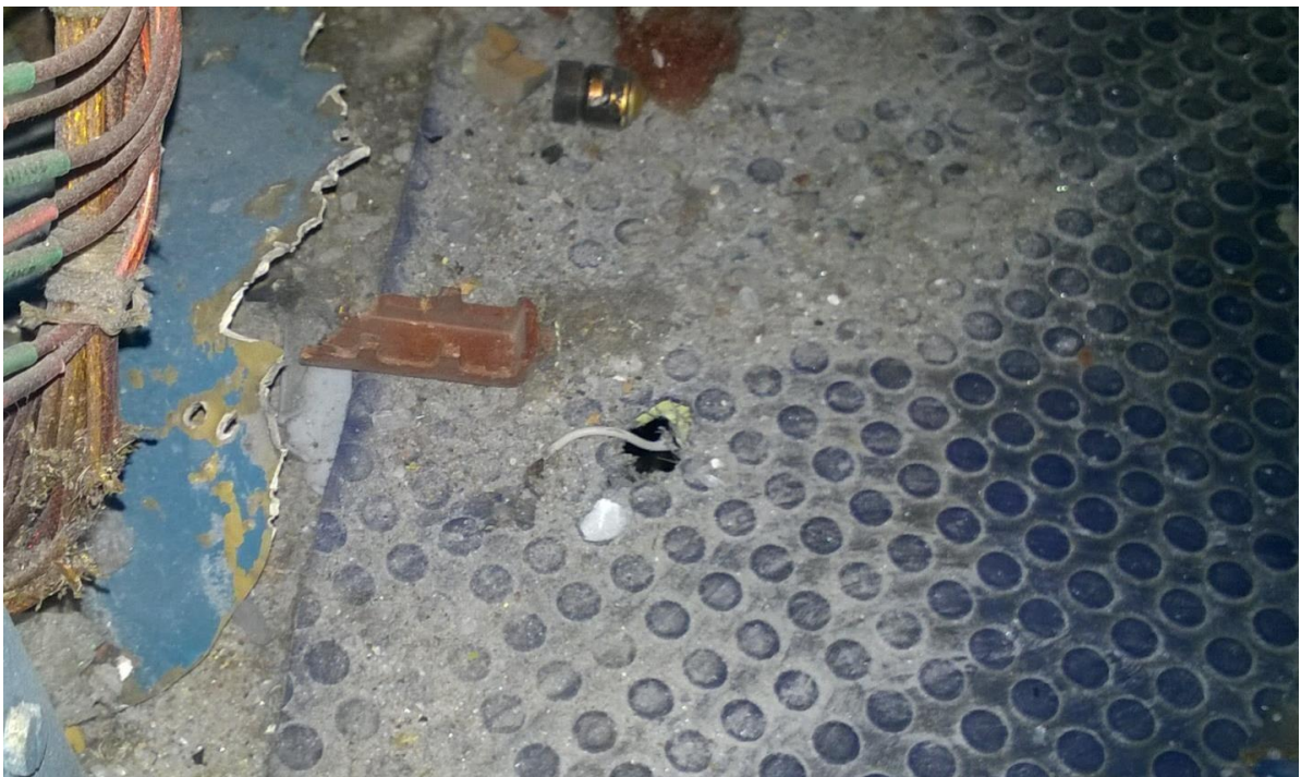
Figure 5.123 - Through-and-through holes in the cockpit floor (starboard)
