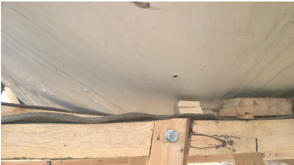
Figure 5.84 - Exit holes and non-penetrating damage
