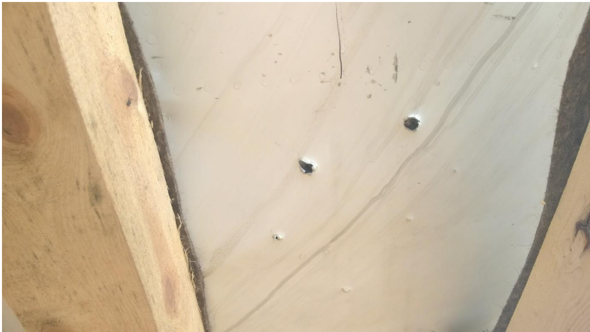
Figure 5.83 - Exit holes and non-penetrating damage
