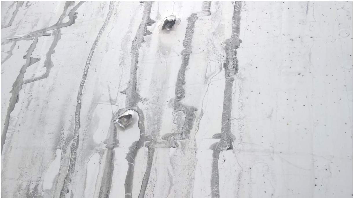
Figure 7.6 - Exit holes on the starboard side
