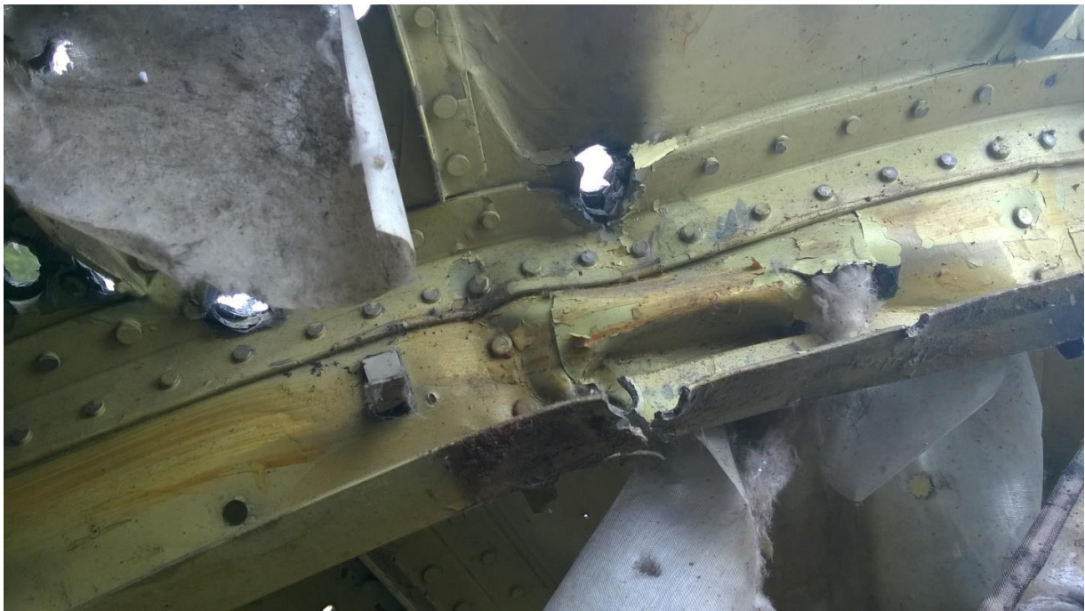
Figure 5.151 - Characteristic view of damage to frames on the left side of the cockpit (punctured L-shaped frame reinforcements). The direction of the motion of the projectiles is transverse to the aircraft structure. There are no through-and-through holes in the frames.
