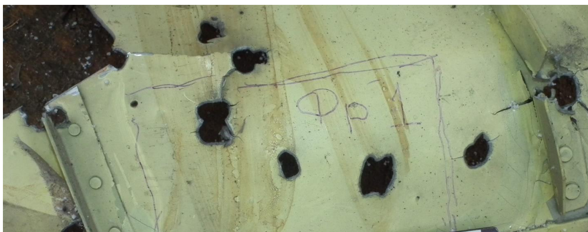
Figure 5.158 - Fragment No. 1 after extraction (close-up, inside view)
