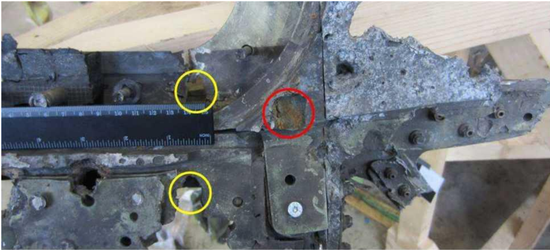
Figure A.2.5 - Example of non-penetrating damage to a glazing frame
