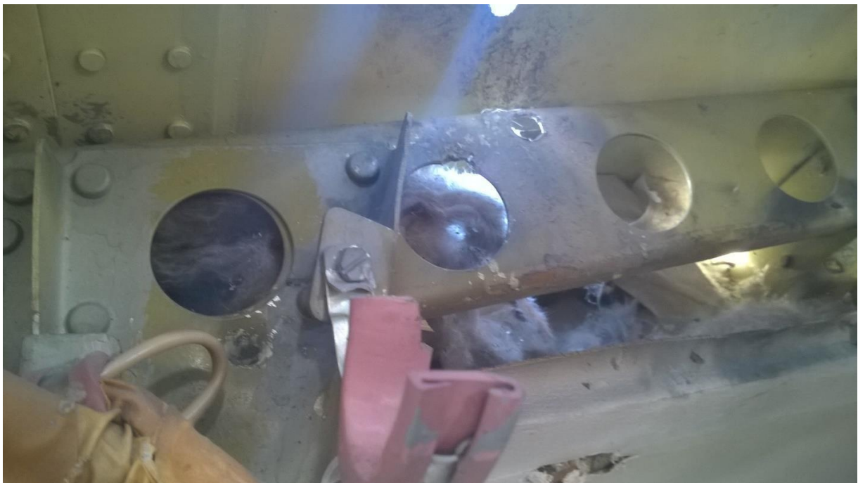
Figure 5.145 - Through-and-through holes in a structural element of the airframe (stringer)
