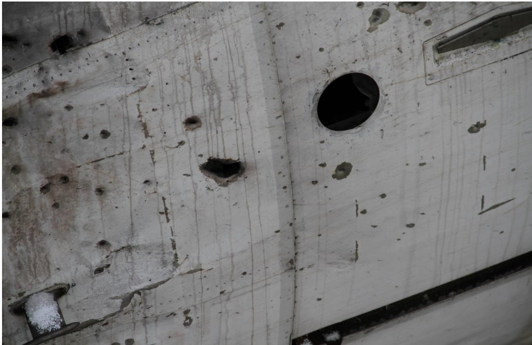
Figure 9.3 – Holes left by second compartment hull fragments on the port side of the target in the area of door L1
