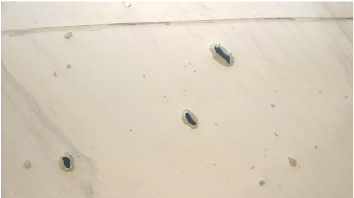
Figure 5.98 - Exit holes and non-penetrating damage
