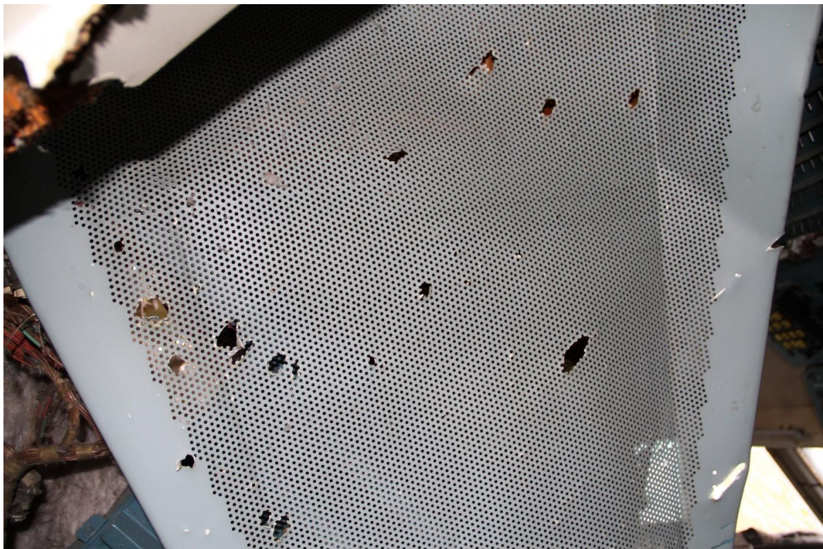
Figure 5.112 - Decorative panel of the cockpit roof
