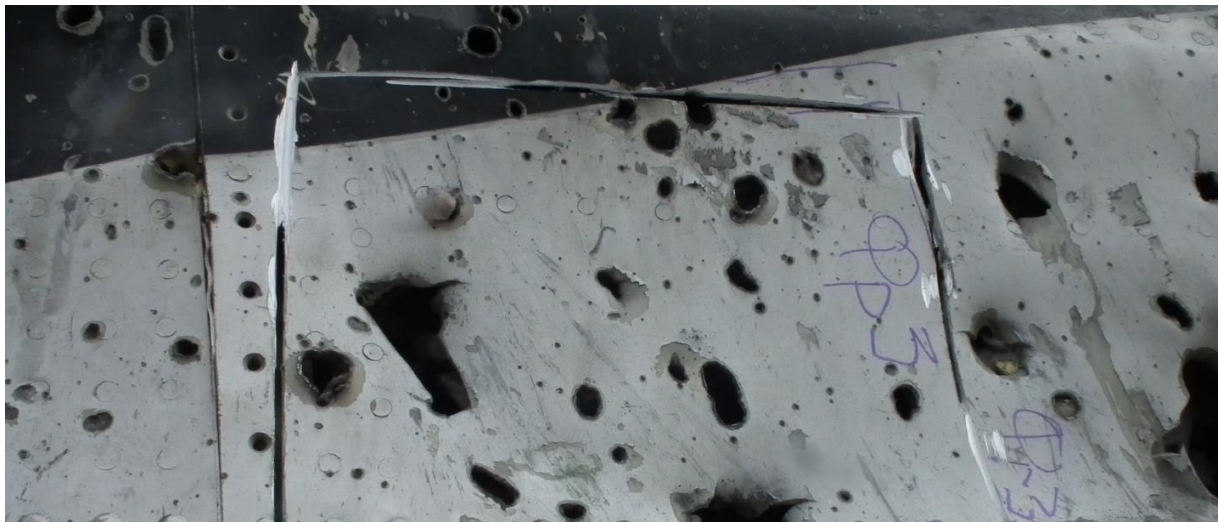
Figure 5.161 - Fragment No. 3 before extraction (external view)
