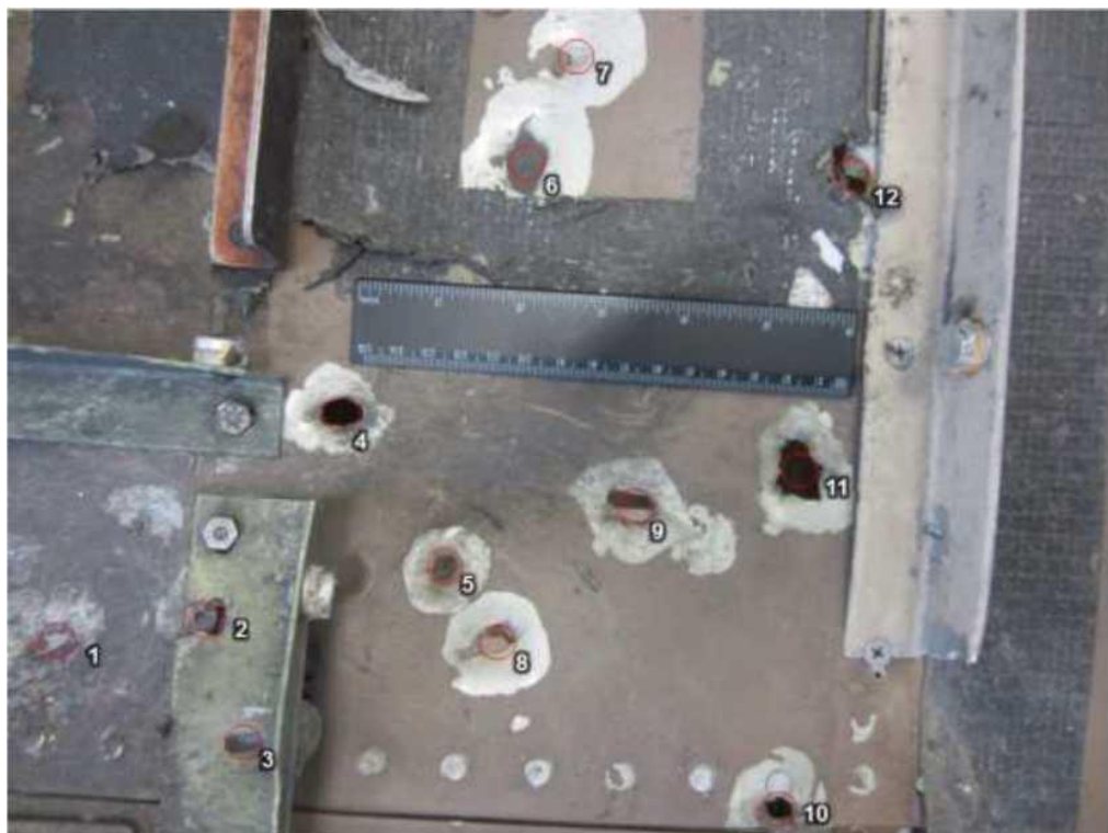
Figure 5.1.48 - Fragmentation damage to cockpit floor to the left of the aircraft commander's seat (along the port side)
