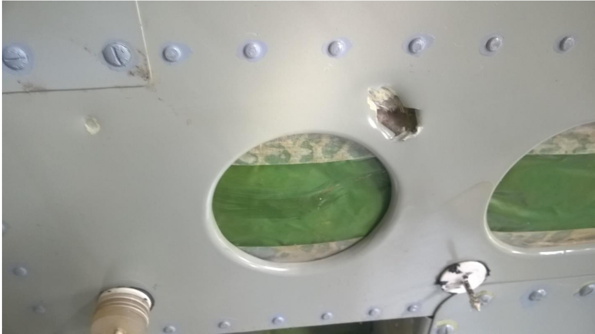
Figure 5.105 - Through-and-through hole in door R1 (inside view)
