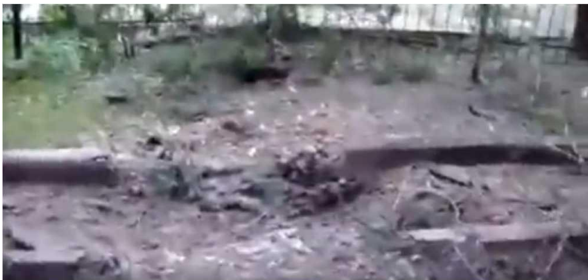
Fig. 14. A sidewalk curbstone hit by a shell between the residential buildings located at 85A Andreyva Linyova Street and 81 Andreyva Linyova Street [17].
