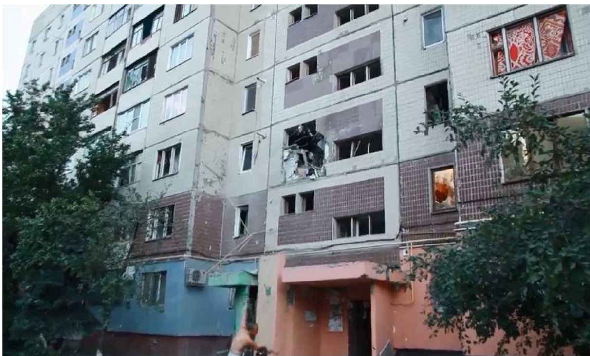
Fig. 10. The hole resulting from the detonation of the shell that hit the northern wall of a multi-storey residential building located at 16 Olkhovsky quarter at the level of the third floor [13].
