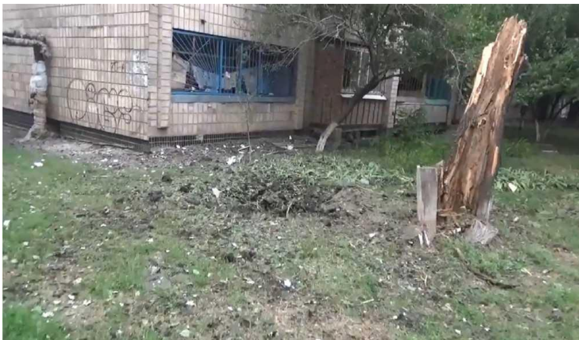
Fig. 13. A crater resulting from the explosion of a shell on the lawn several metres from the south-northern corner of the multi-storey residential building located at 79A Andreyva Linyova Street [16].
