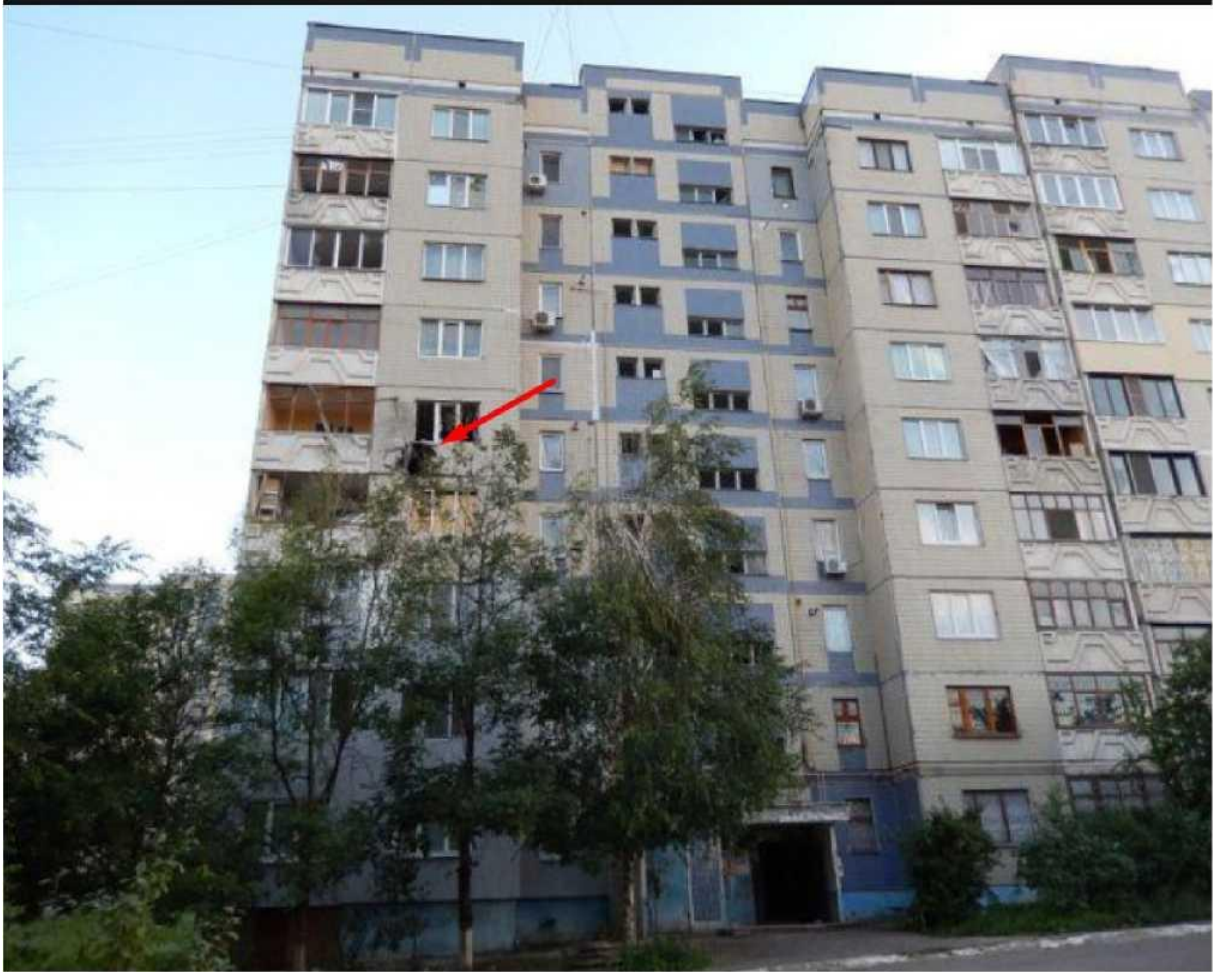
Fig. 8. The northern wall of a multi-storey residential building located at 6 Stepnoy quarter hit by a shell at the level of the fifth floor [11].
