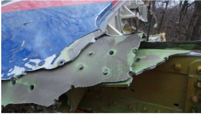
1 2 Figure 62 – Tensile overstress fracture at the outside of the lower left door corner of 3 door 3R (source: DSB) 4
