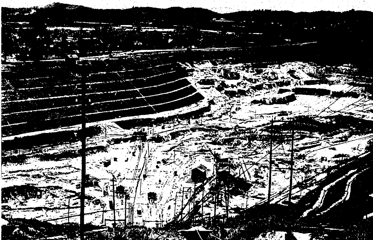
Open Cast Tin Mine showing broken down terraces in process of restoration.
