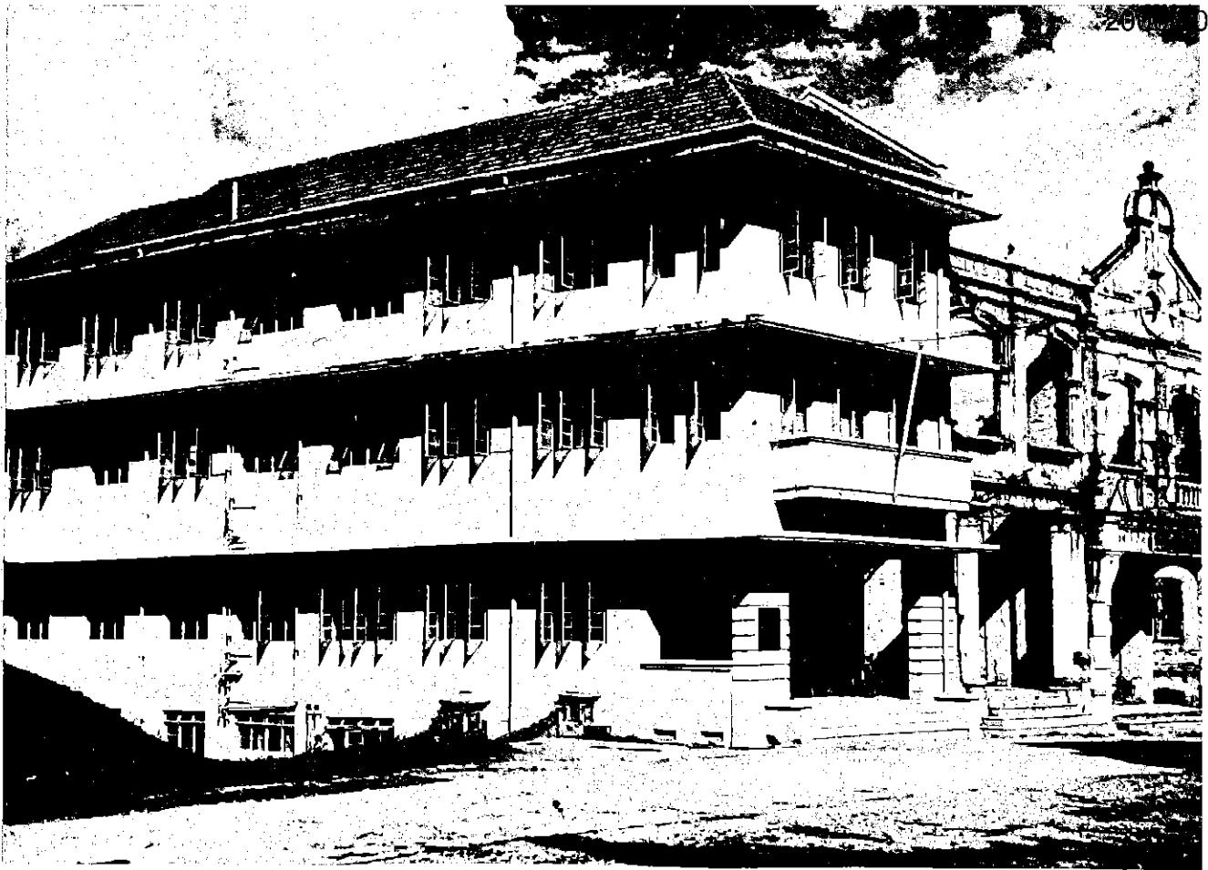
F.M.S. Chamber of Mines building restored.
