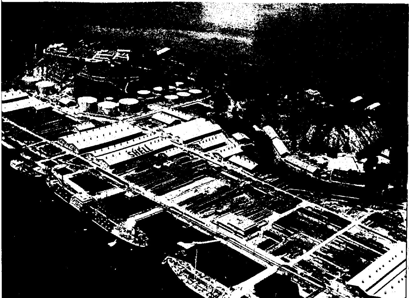
Shell Company's installations after rehabilitation.
