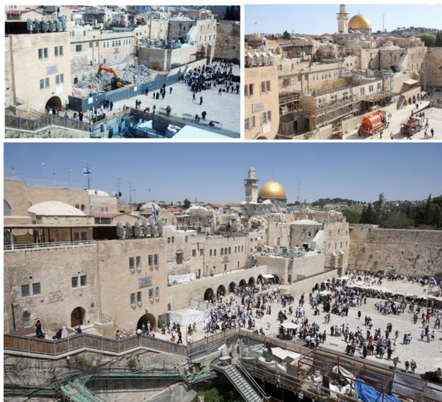
Demolitions for the construction of Beit Strauss on Muslim Waqf real-estate, 2013-2016
