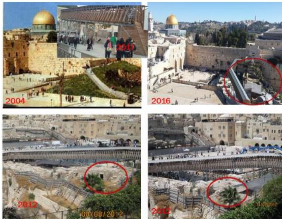
Figure 81: Systematic demolitions of historic room, walls and continued excavations and constructions at the MGP, 2004 through 2017.
