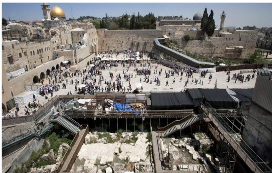
Beit Haliba Project at the site of the historic Magharbeh Quarter
