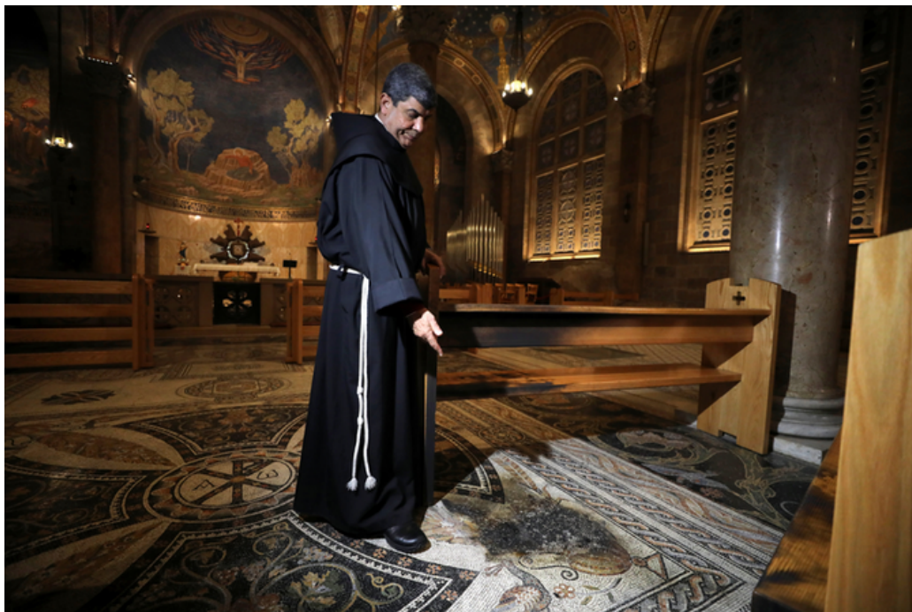
Franciscan Father Ibrahim Faltas inspects the damage after a man tried to set fire to Gethsemane Church in Jerusalem, Dec. 4, 2020. (Reuters)
