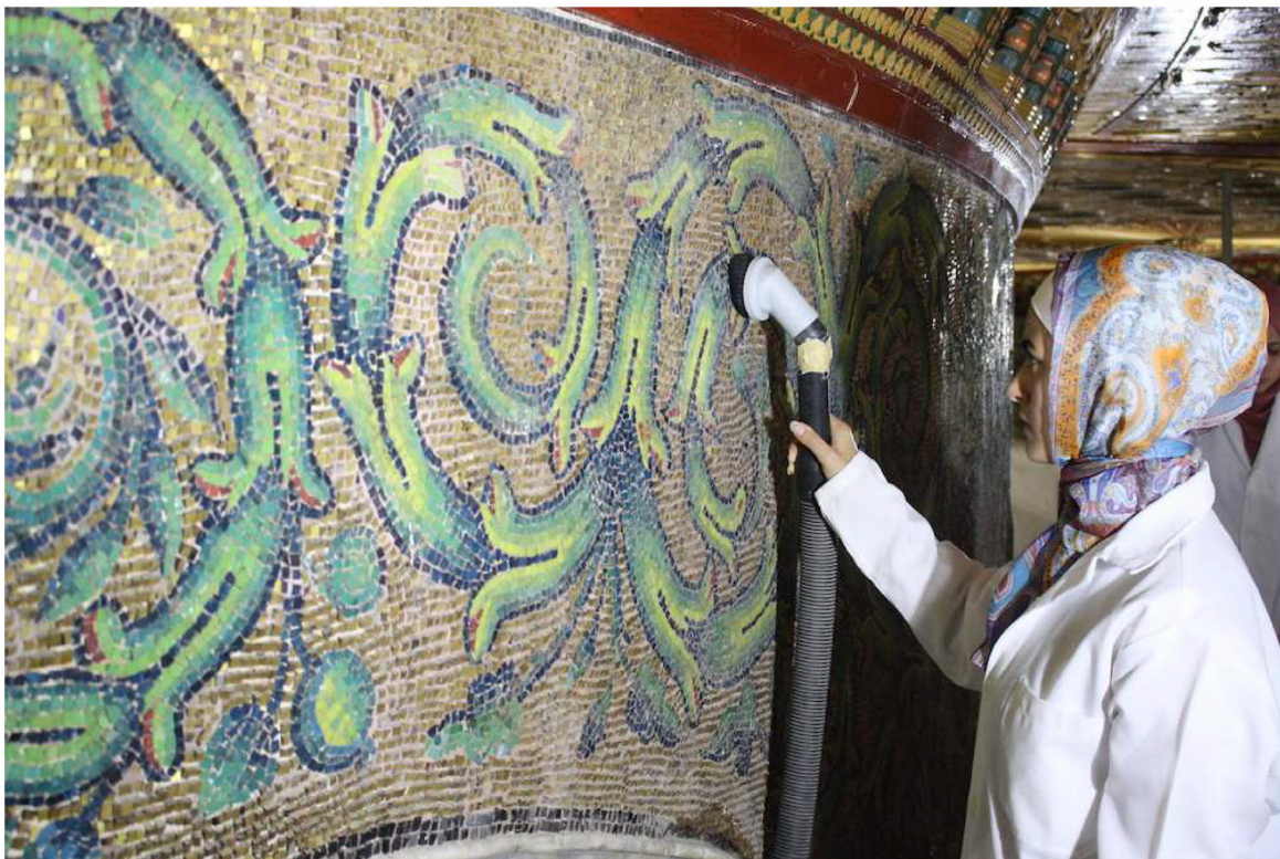
An engineer dry cleaning the mosaic painting after renovating some impaired pieces. (Supplied)
