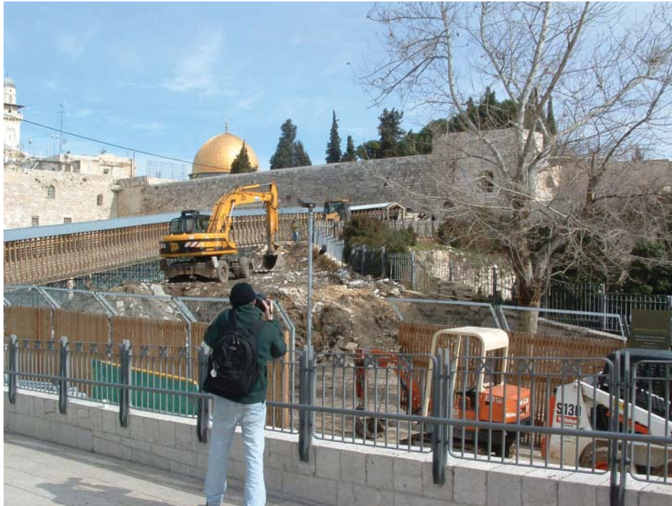
FIGURE 2 Preparations for excavation on the Mughrabi ramp, 2007.
