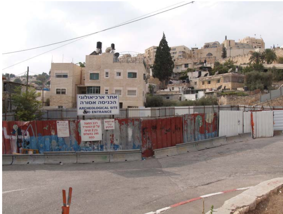
FIGURE 7 Excavations at the Giv'ati parking lot in Wadi Hilweh, Silwan.
