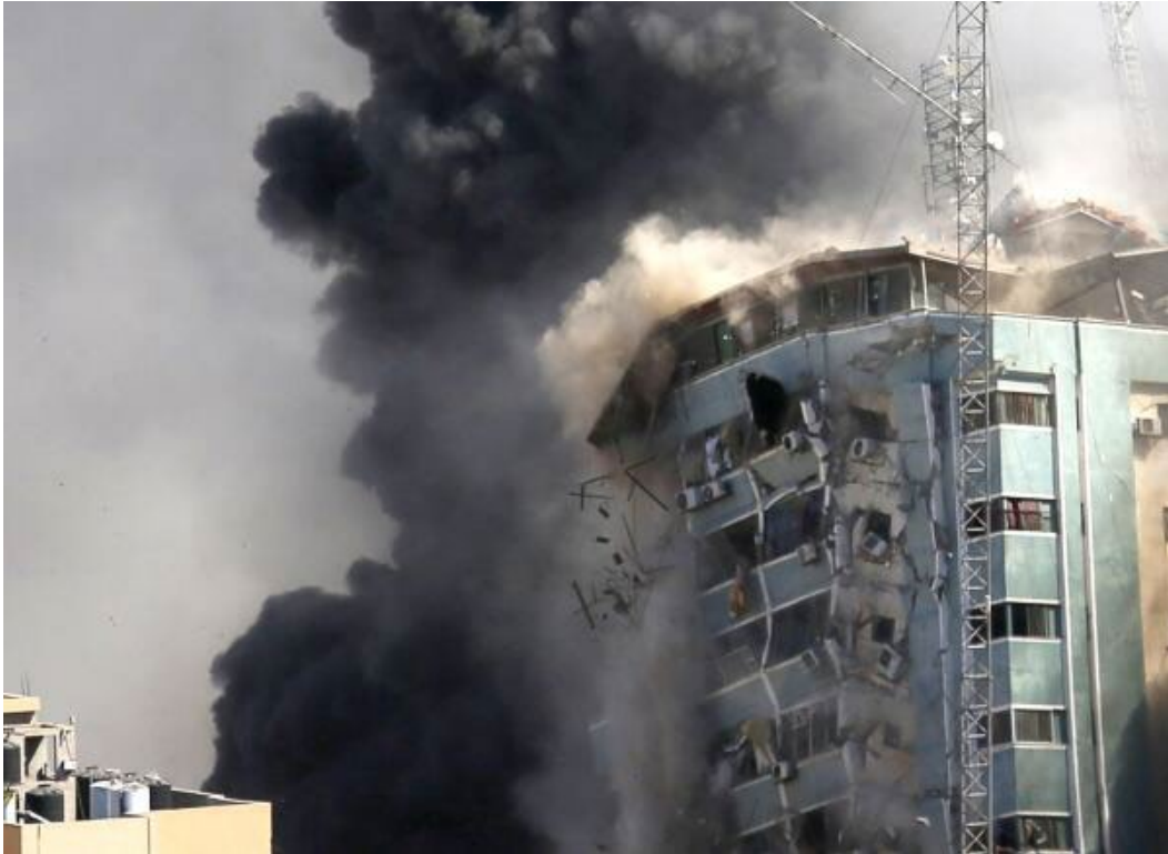
Figure 2.38: The building housing the offices of the Associated Press and other media in Gaza City collapses after it was hit by an Israeli airstrike, 15 May 2021 711
