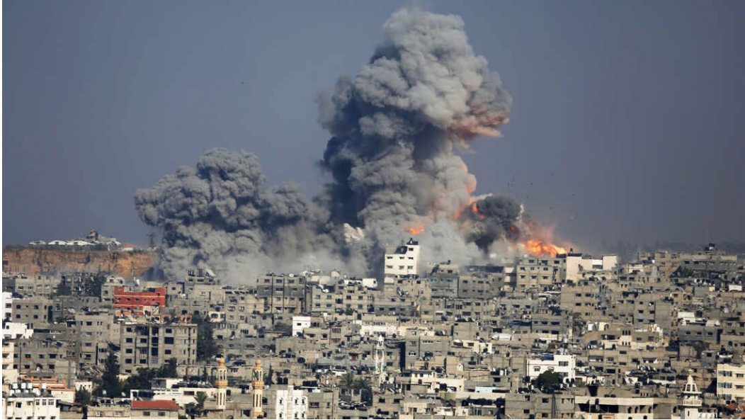
Figure 2.22: Smoke and fire rise from the explosion at the Gaza power plant, 29 July 2014 372
