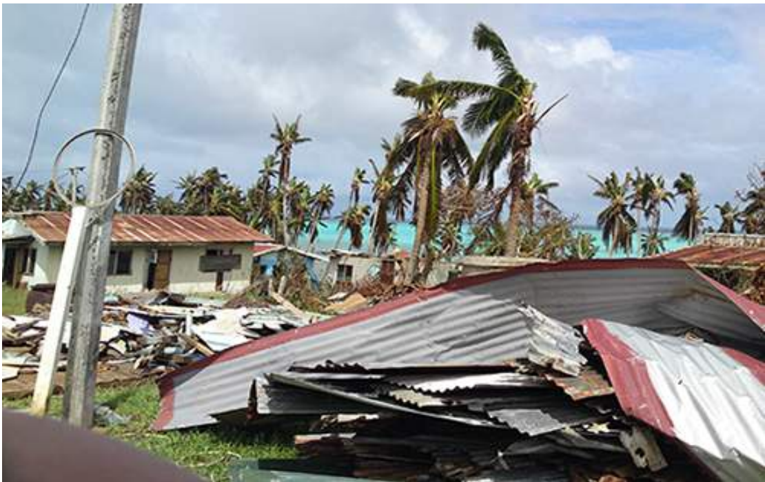
Figure 10. Photograph of damage caused by Cyclone Pat - February 2010
