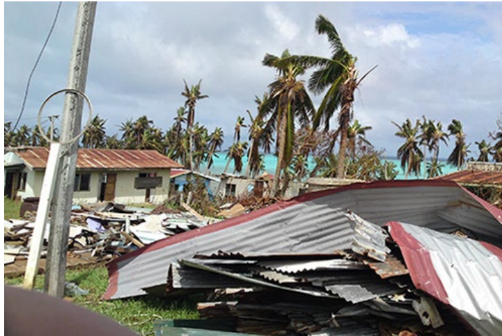
Picture 1. Example of damage caused by Tropical Cyclone Pat, February 2010.
