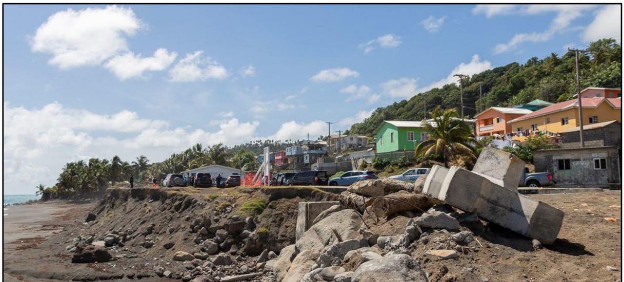
Coastal Erosion at Sandy Bay in SVG
