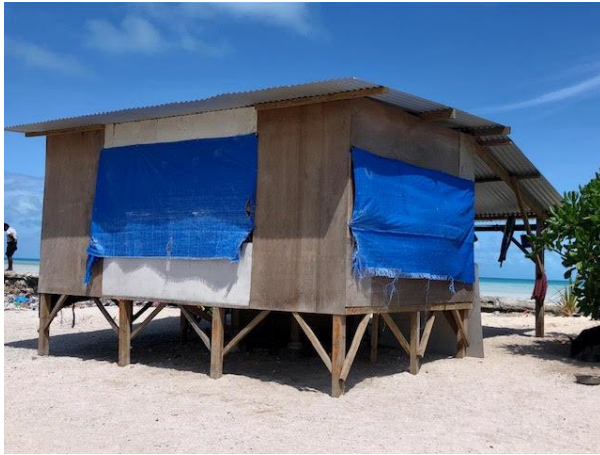
Elevated houses in Tebikeinano
