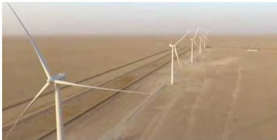
Figure (5-3) :Shagaya (phase I) 10 MW wind turbines, total of 5 wind turbines each of 2 MW.
