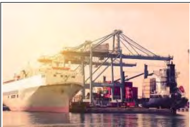
Figure 1-33: Shuwaikh seaport. (Source: Kuwait Ports Authority website)
