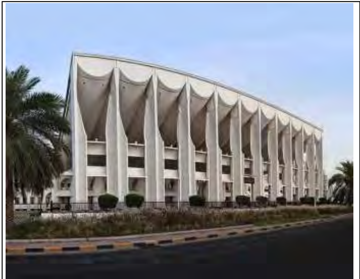
Figure 1-17: Kuwait National Assembly building. (Source: KNA official website)
