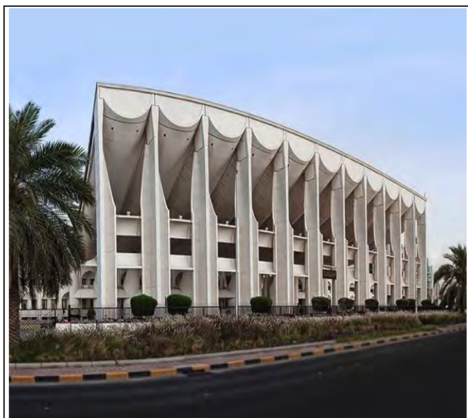
Figure 1-37: Kuwait National Assembly building.
