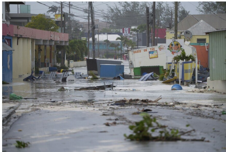
Figure 2: Impassable Road at Hastings Barbados following Hurricane Beryl 5
