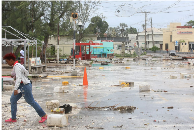
Figure 1: Impassable Road at Oistins Barbados following Hurricane Beryl 4
