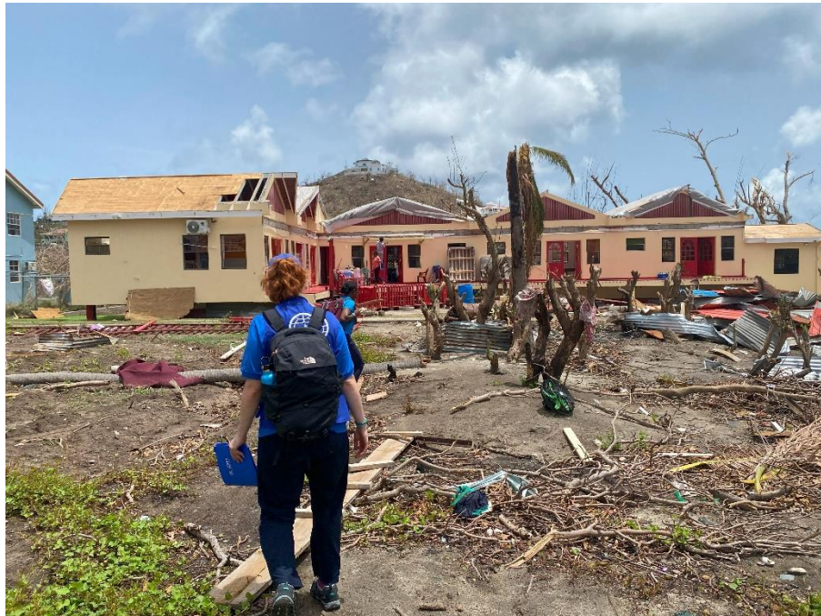
FIGURE 9: SUNSET HOTEL IS AN INFORMAL POP-UP SHELTER IN CARRIACOU, CURRENTLY HOUSING AT LEAST 9 PEOPLE. THERE ARE LARGE SECTIONS OF THE ROOF MISSING, RESIDENTS ARE CRAMPED INTO TWO ROOMS, AND MOSQUITOS ARE BECOMING A SIGNIFICANT PROBLEM. PHOTO: JOLENE MUIR, OCHA
