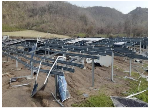
Complete detachment of the modules from rails
