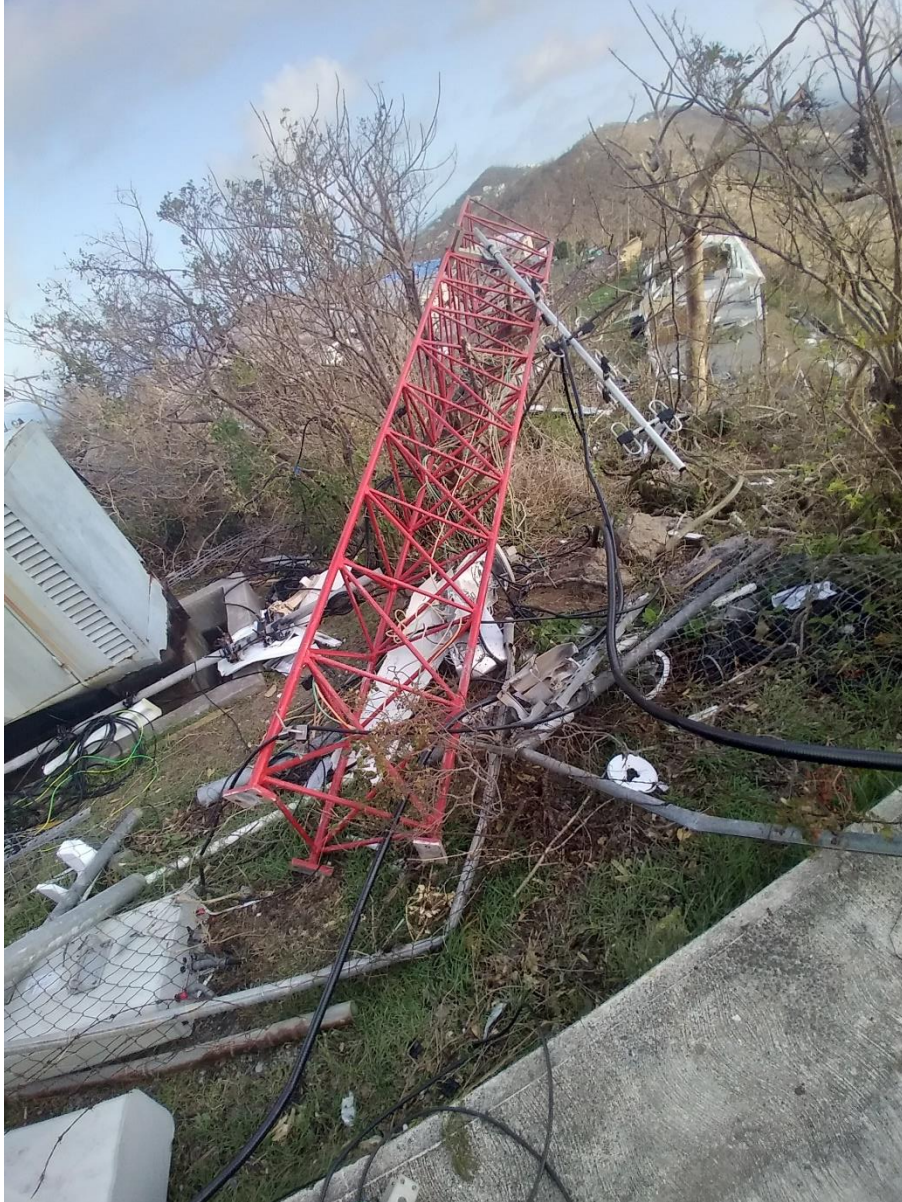
Broken tower at Belair, Carriacou
