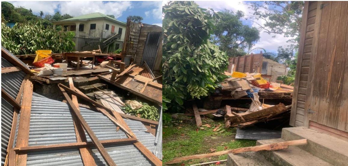
Figure 10: Pictures showing flatten boucan and watchman house at Mt. Reuil Estate
