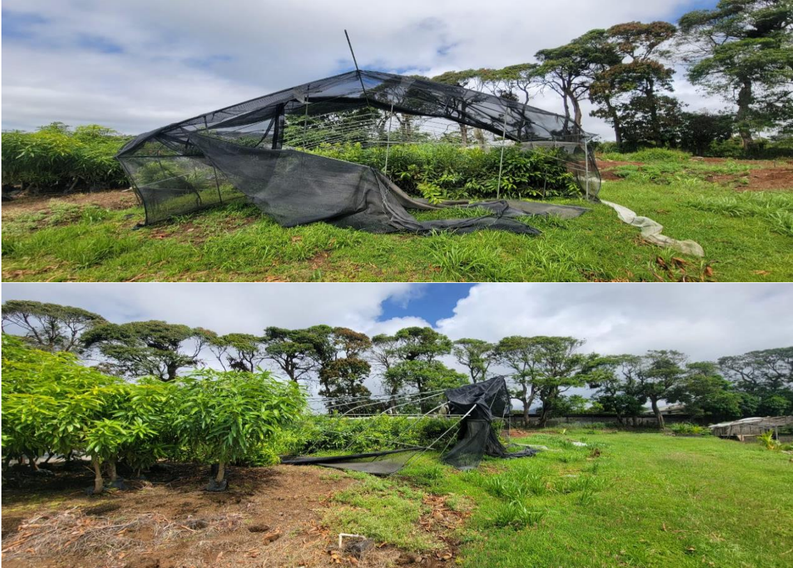
Figure 8: Pictures and damaged greenhouses at Mirabeau Station
