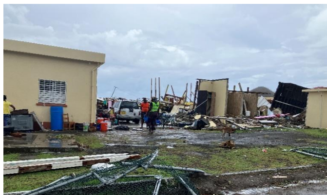
FIGURE 11: ONLY THE LIBRARY AND ONE BATHROOM REMAIN AT THE DOVER PRIMARY SCHOOL IN CARRIACOU. PHOTO: LISA MCCLEAN TROTMAN, UNICEF
