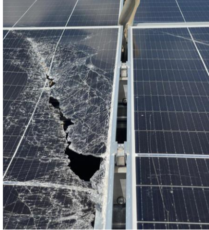
Complete detachment of the modules from rails
