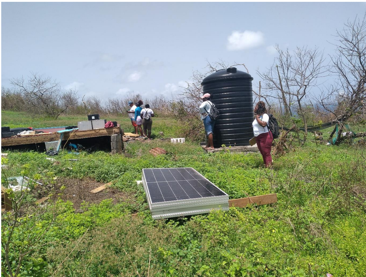
One of 13 fishermen camp houses destroyed at Isle De Rhonde
