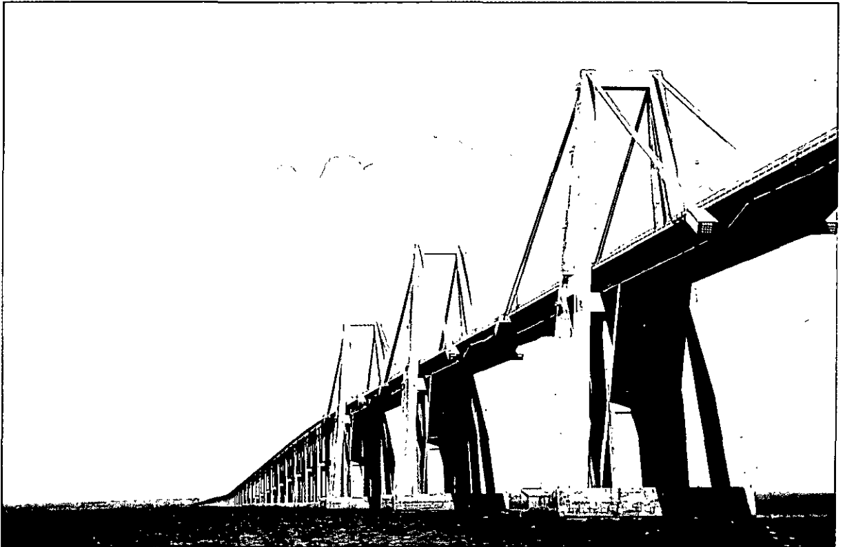
Figure 19: THE MARACAIBO BRIDGE
