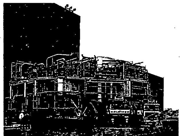
Transportation of an outfitted deck from the main assembly hall to the yard.
