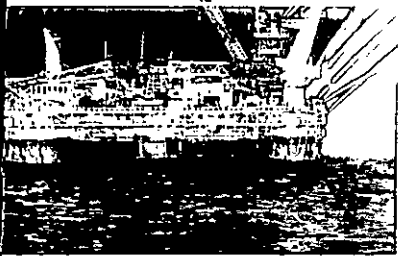
MSV, Stadive Seaforth Maritime/Shell Expro, U.K. November 1982
