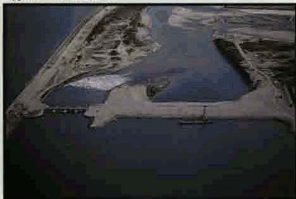
Bypass weir and dam
